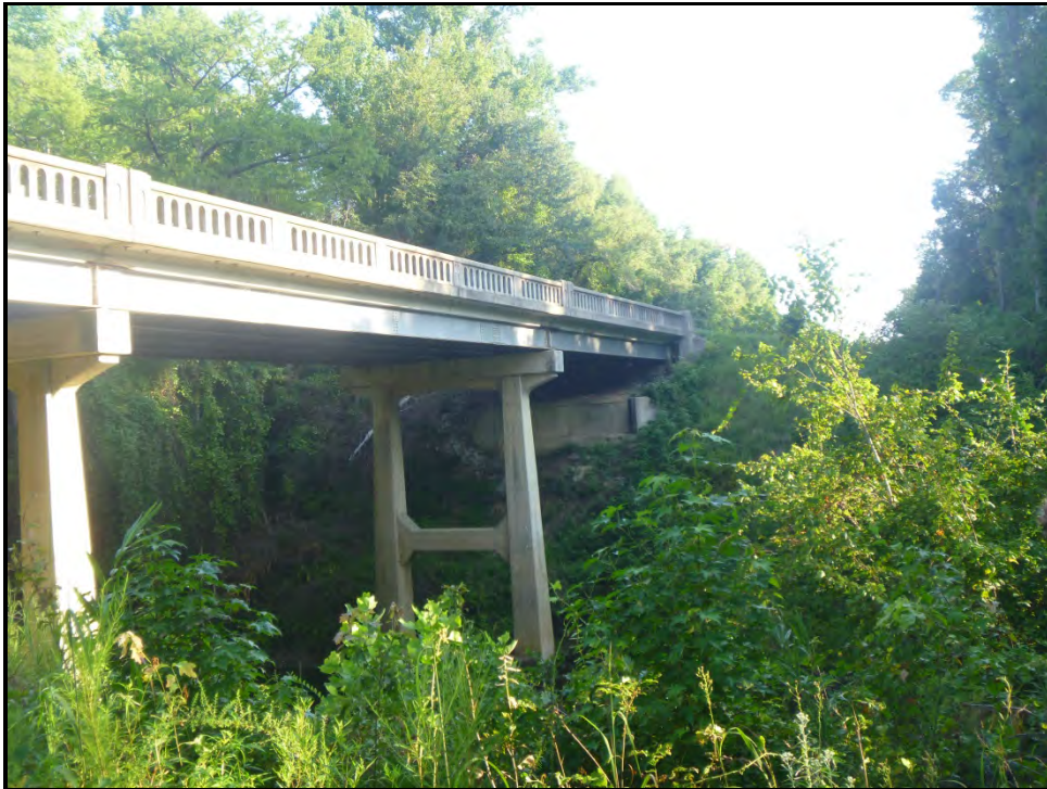
Figure 8: Bridge 60, facing North from Southeast Quadrant of APE.
