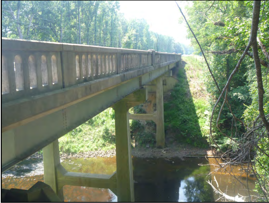
Figure 15: Bridge 60, facing Southwest from Northwest Quadrant of APE.
