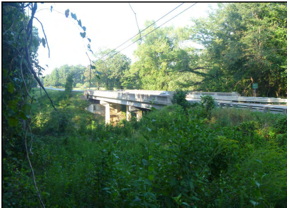
Figure 10: Bridge 60, facing West from Northeast Quadrant of APE.
