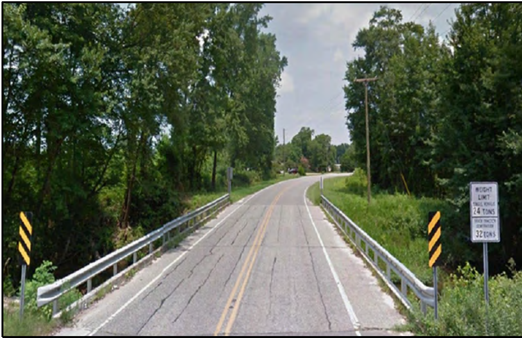
Bridge No. 434 looking North
