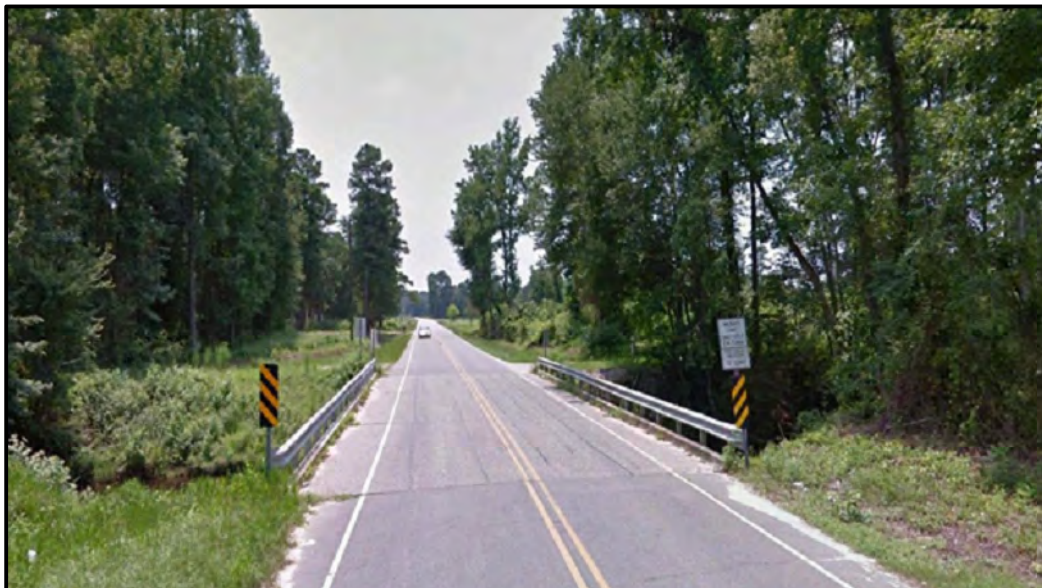
Bridge No. 434 looking South
