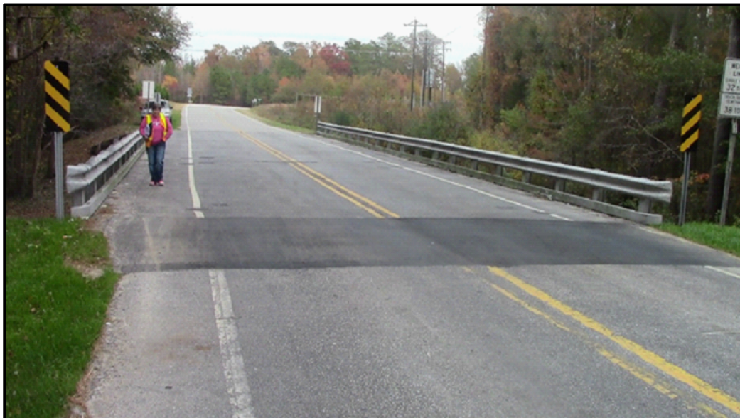
Bridge No. 72 looking North
