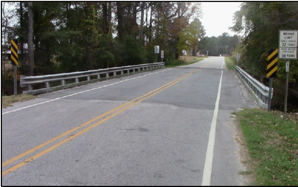
Bridge No. 72 looking South
