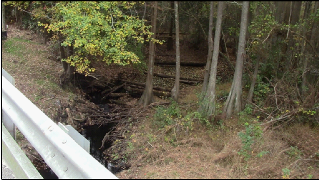
View from Bridge No. 72 Looking West
