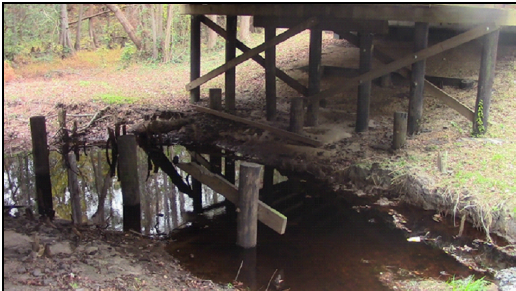
View under Bridge No. 72
