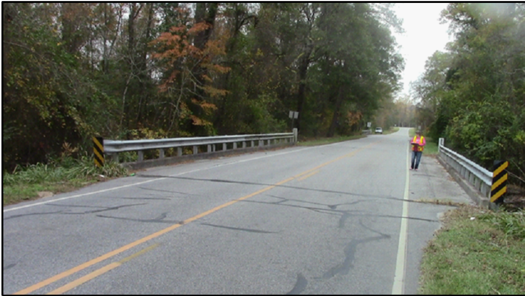
Bridge No. 400 looking Southwest
