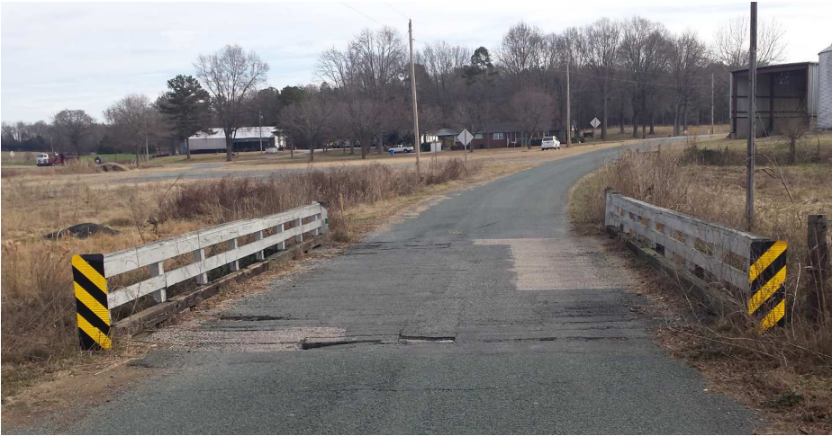
Picture 1: Looking eastbound along Gullede Parker Road from Bridge No. 448
