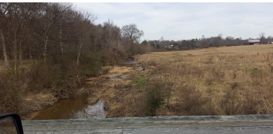
Picture 4: Looking north along Buffalo Creek from Bridge No. 448
