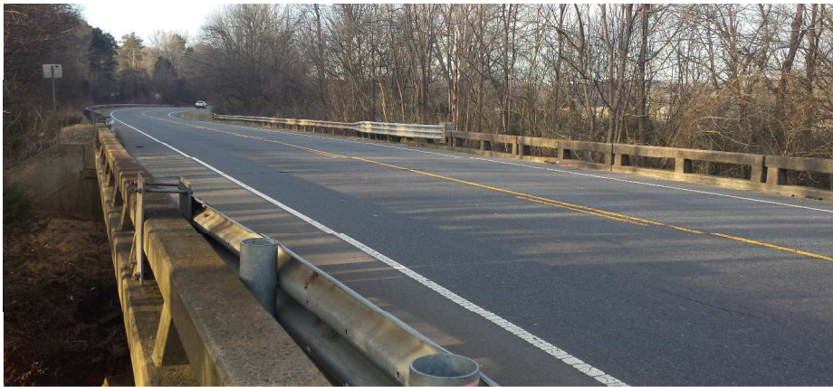
Picture 2: Looking south along US 601 from Bridge No. 71.
