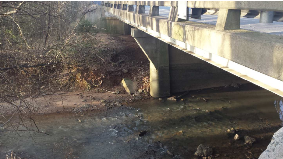
Picture 6: Looking at Clear Creek from the road shoulder on US 601.
