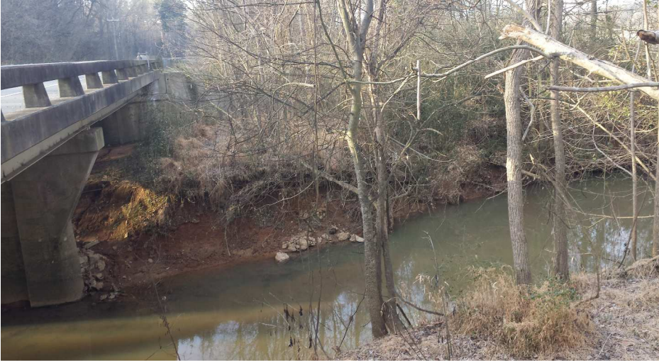
Picture 5: Looking at Clear Creek from the road shoulder on US 601.
