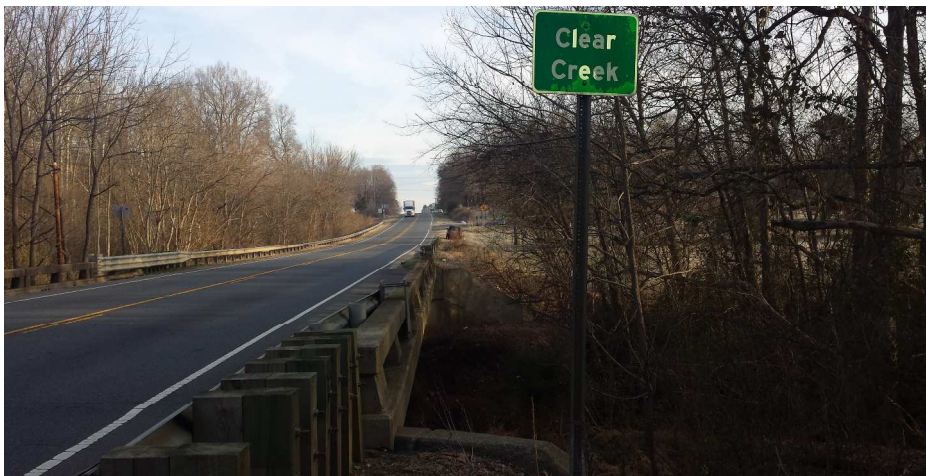
Picture 4: Looking north along US 601.
