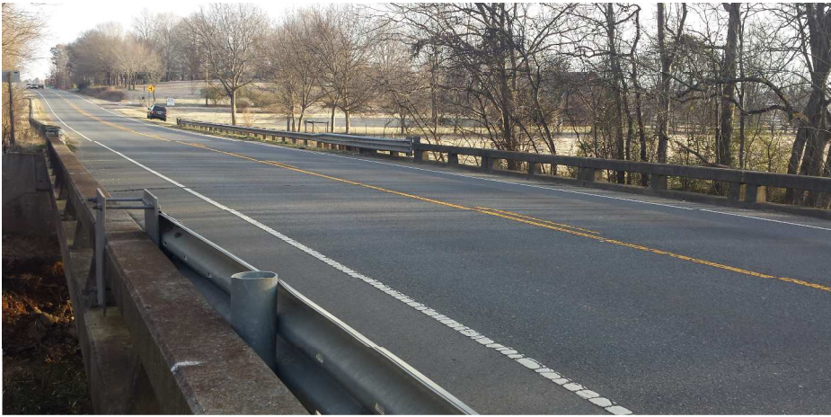
Picture 1: Looking north along US 601 from Bridge No. 71.
