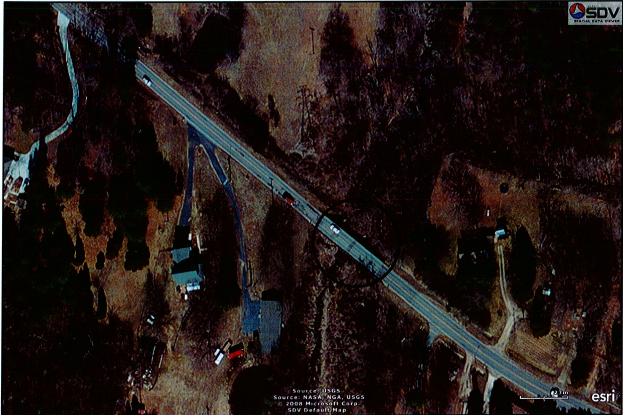
Figure 1. Bridge 53 over Cold Water Creek.
