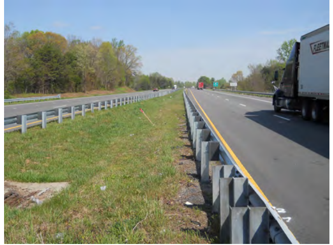
US 220 Approach Roadway Looking North
