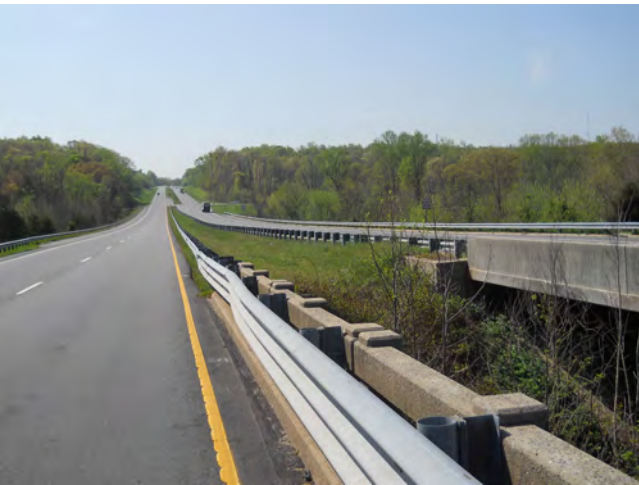
US 220 Bridge Structure Looking South
