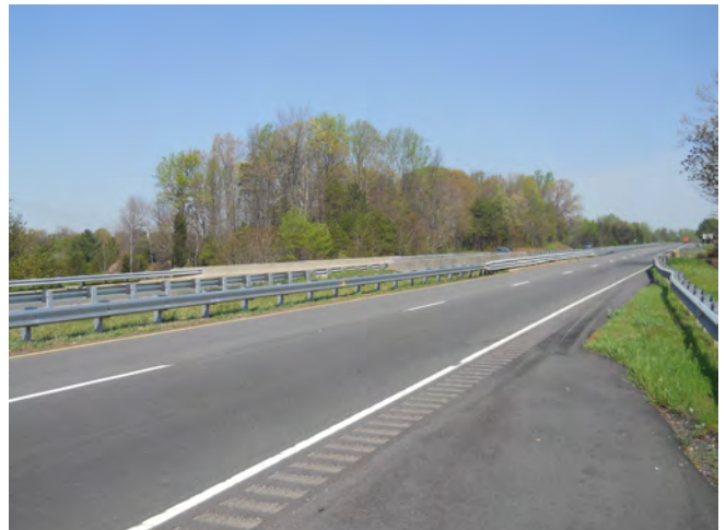
US 220 Approach Roadway Looking North
