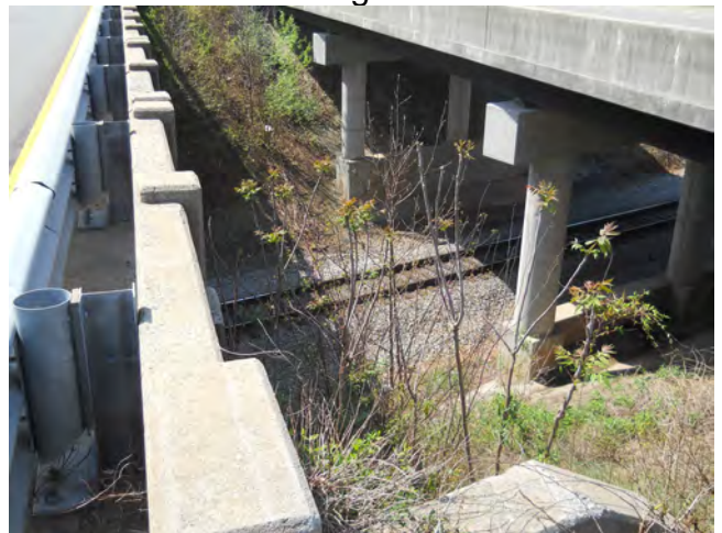
US 220 Bridge Substructure Over Norfolk Southern Railroad
