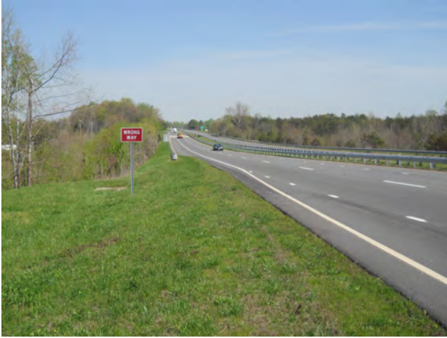
US 220 End of Bridge Looking North
