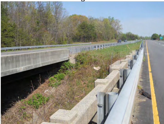
US 220 Bridge Structure Looking North
