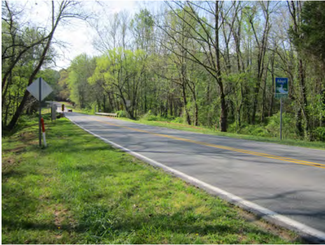
SR 2136 (Fleming Road) Approach Roadway Looking North
