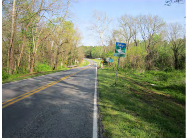
SR 2136 (Fleming Road) Approach Roadway Looking South
