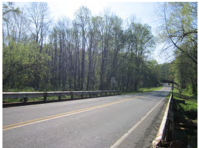
SR 2136 (Fleming Road) Bridge Looking North
