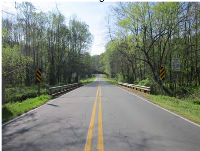
SR 2136 (Fleming Road) Bridge Approach Looking North
