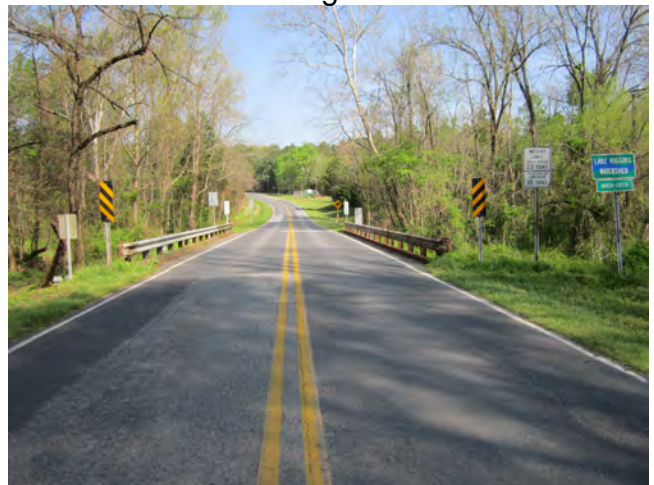
SR 2136 (Fleming Road) Bridge Approach Looking South
