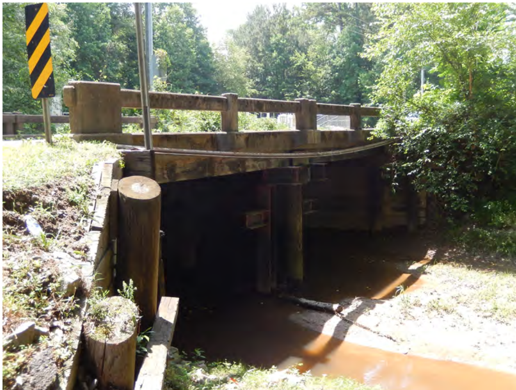
East Face of Bridge No. 247
