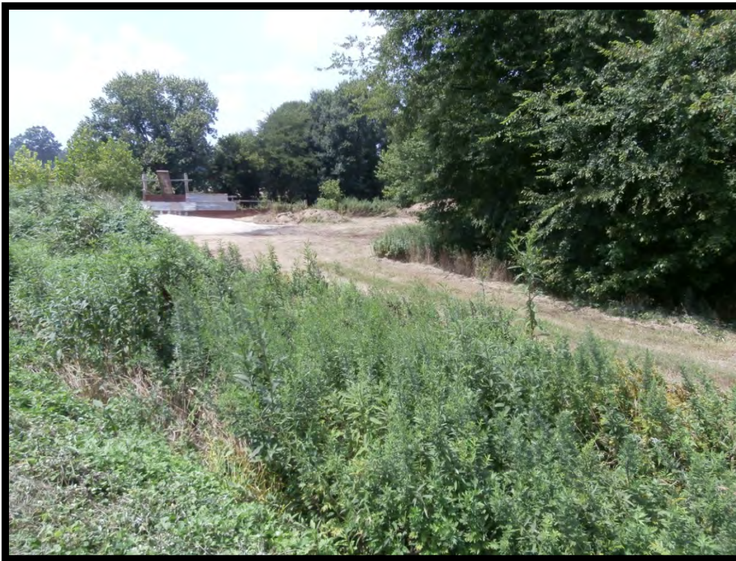
View of Disturbed Area with Sand Dredging Operation Area, Along the East Side of Muddy Creek and North of Hampton Road, Looking North-Northwest.
