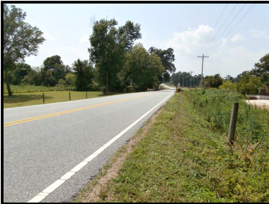
View of Bridge Over Muddy Creek, Looking West.
