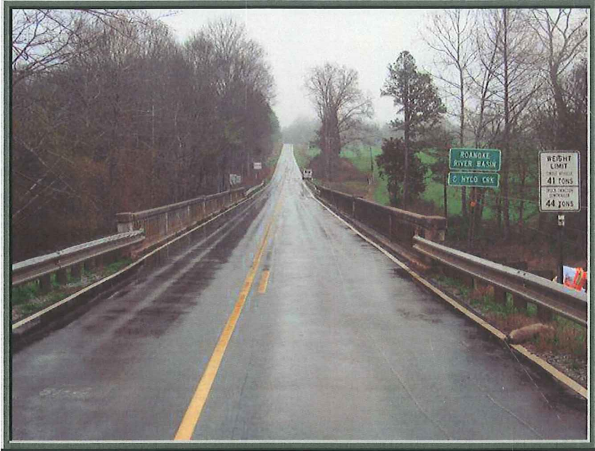
Eastbound Approach Bridge No. 11
