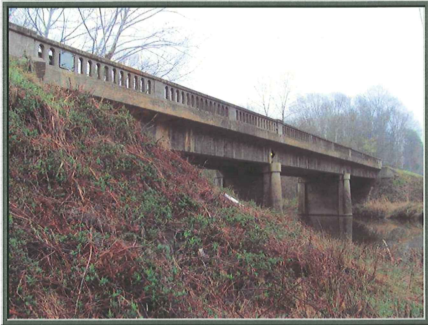
South Face of Bridge No. 11
