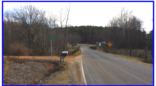
Looking east at Bridge No. 291 on Old N.C. 90
