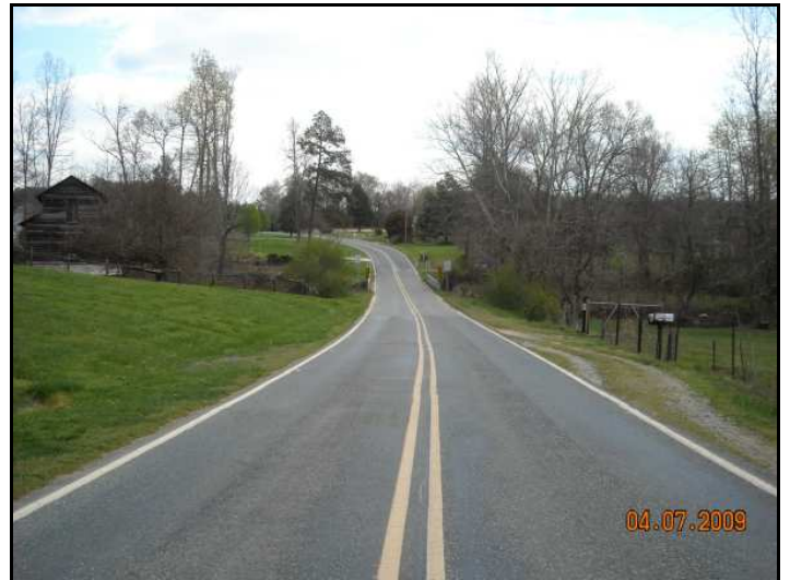
Bridge No. 64 on SR 1912 – View to the East
