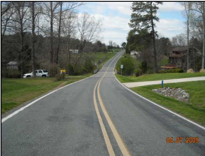
Bridge No. 64 on SR 1912 – View to the West
