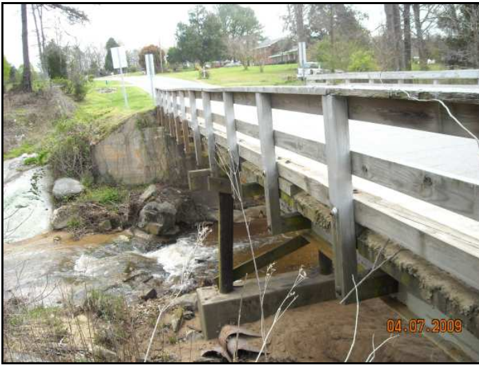
Bridge No. 64 on SR 1912 – Left Bridge Face
