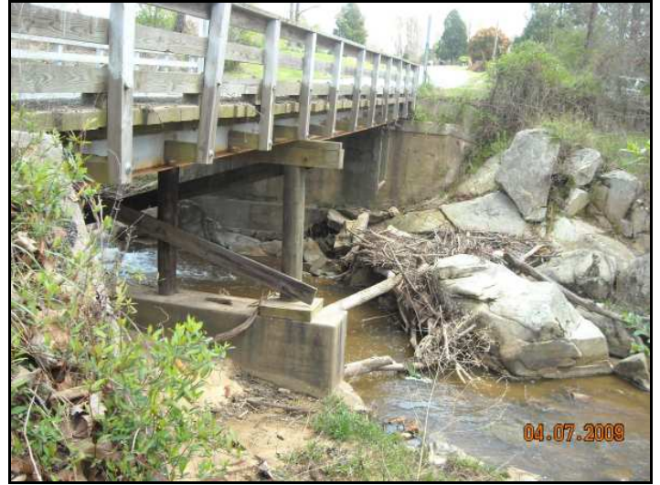
Bridge No. 64 on SR 1912 – Right Bridge Face
