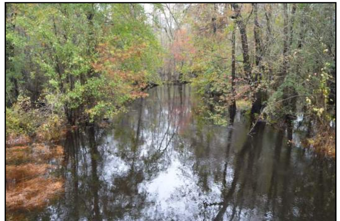
Bridge No. 172 facing North towards South River
