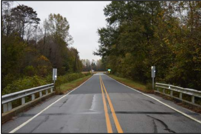
Bridge No. 171 approach facing East
