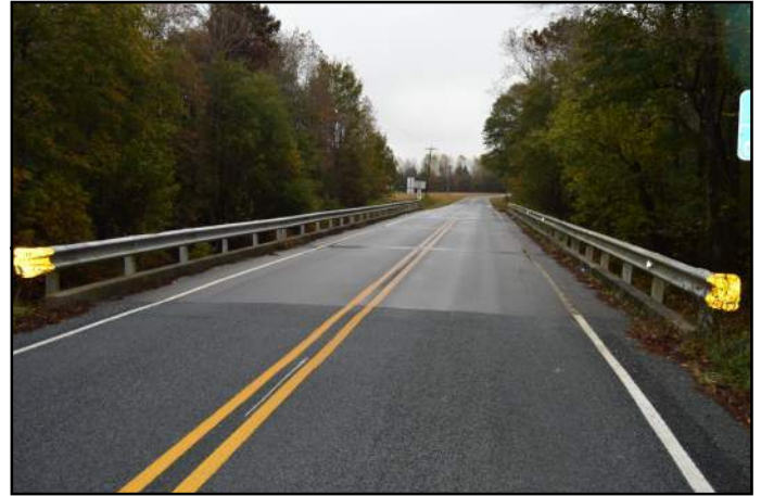
Bridge No. 172 approach facing East
