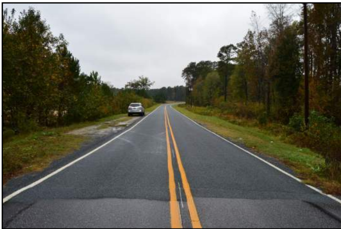
Bridge No. 171 facing West
