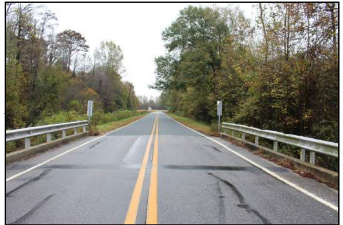
Bridge No. 172 approach facing West
