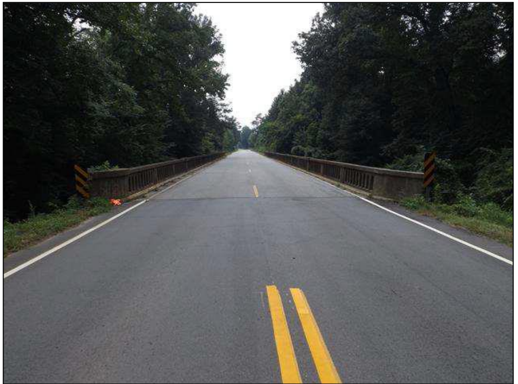
Bridge No. 29 over Little Fishing Creek Looking west
