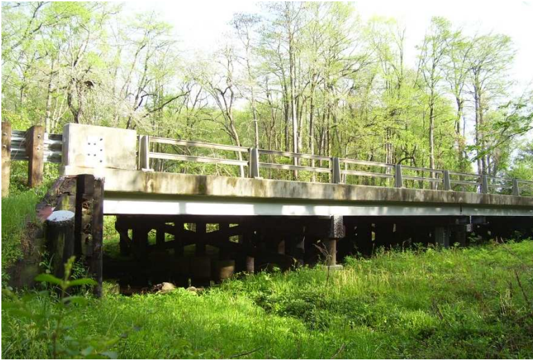
East Face of Bridge
