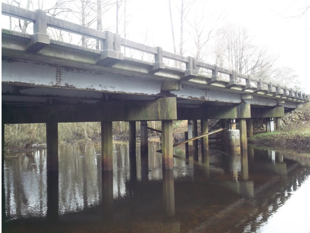
RIGHT SIDE OF BRIDGE NO. 56, FACING WEST
