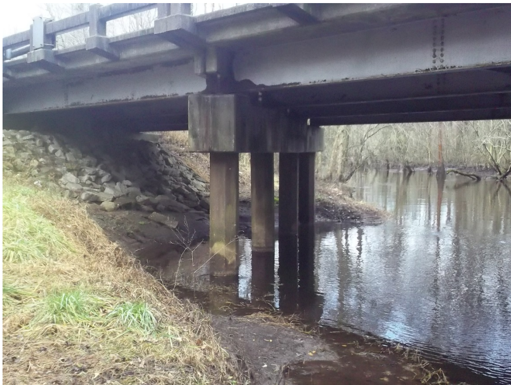
RIGHT SIDE OF BRIDGE NO. 56, FACING EAST
