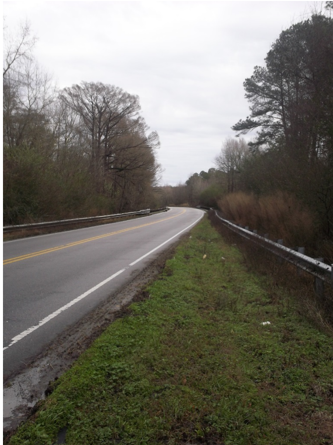
FROM EAST, VIEW OF BRIDGE NO. 56
