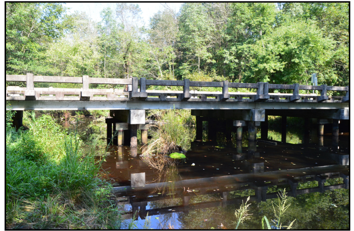
East side of Bridge No. 123
