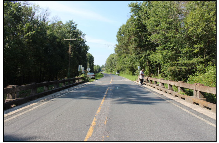
Bridge No. 123 facing SW toward NC 904
