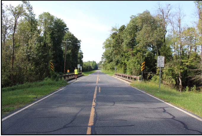
Bridge No. 121 facing SW toward NC 904
