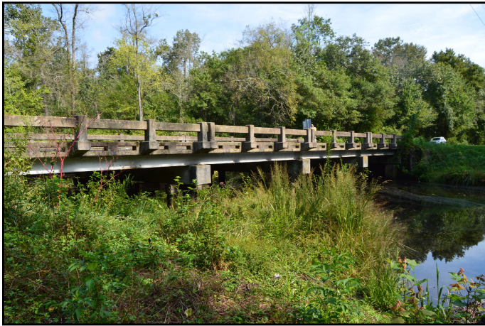
East side of Bridge No. 121
