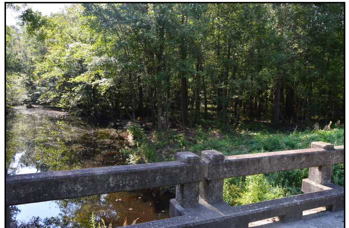
Ashpole Swamp west side of Bridge No. 123
