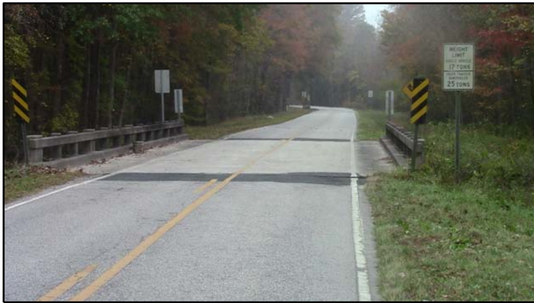
South view from Bridge Nos. 228 and 226
