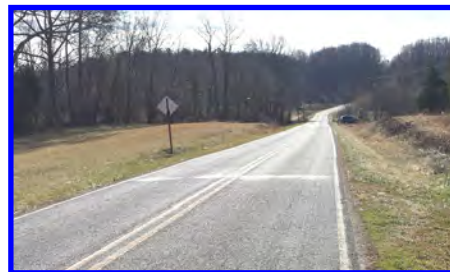
Looking south on Paul Payne Store Road at Bridge No. 130
