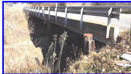
Bridge No. 130 over Elk Shoals Creek
