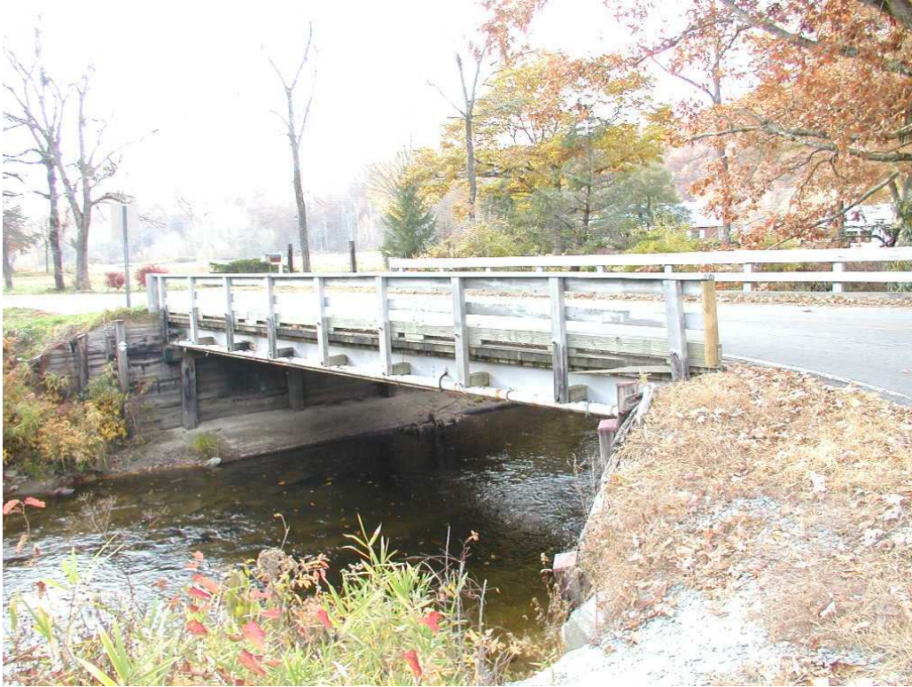
South Face of Bridge
