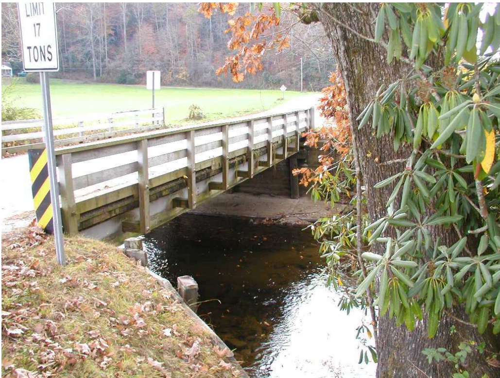
North Face of Bridge
