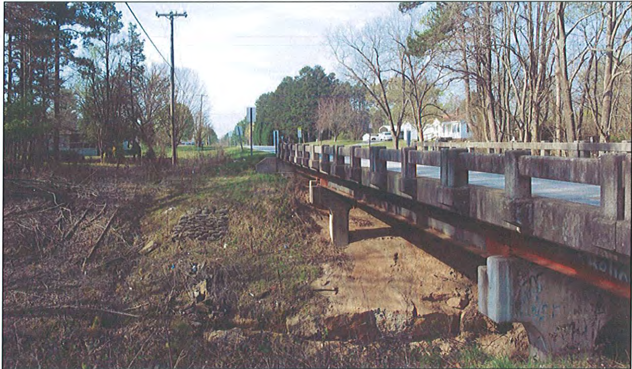
Bridge No. 66, Hurley School Road, Rowan County, facing southwest.
