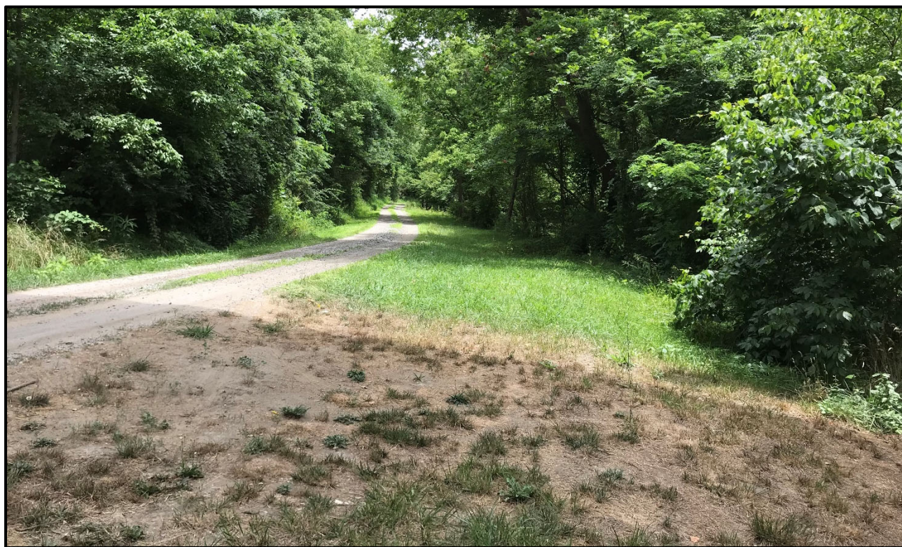
Figure 7. General view of the sewage pipeline in the floodplain looking east from under the bridges.
