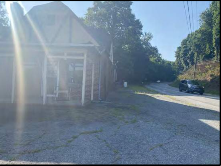
View of Survey Area (Facing Approximately Southeast)
