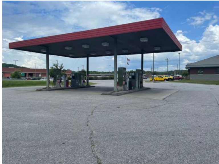
View facing southeast from the western corner of the Project Study Area, depicting the fuel islands, the fuel canopy, and the NCDOT office building.
