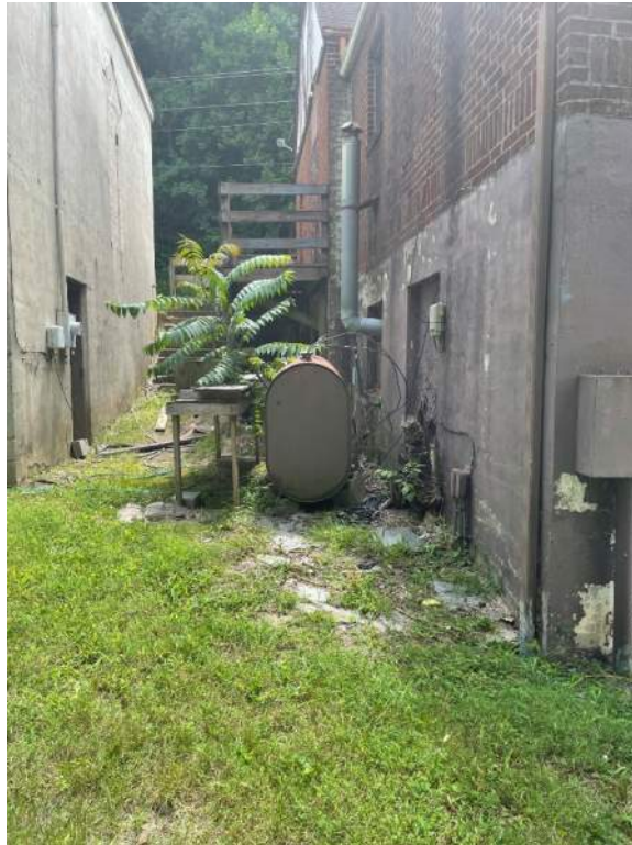
View facing southwest from the eastern portion of the parcel, depicting an approximately 275-gallon heating oil AST located outside of the Project Study Area between the apparent storefront and the eastern adjacent building.
