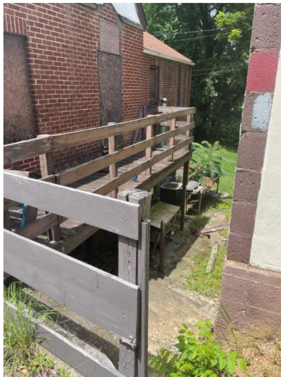
View facing east from the southwestern portion of the Project Study Area along NC 115, depicting the area between the apparent storefront and the adjacent eastern building outside of the Project Study Area.
