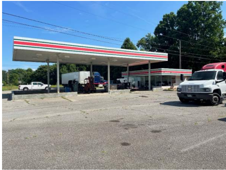
View facing north from the southwestern corner of the Project Study Area displaying inactive fuel islands and an inactive convenience store.
