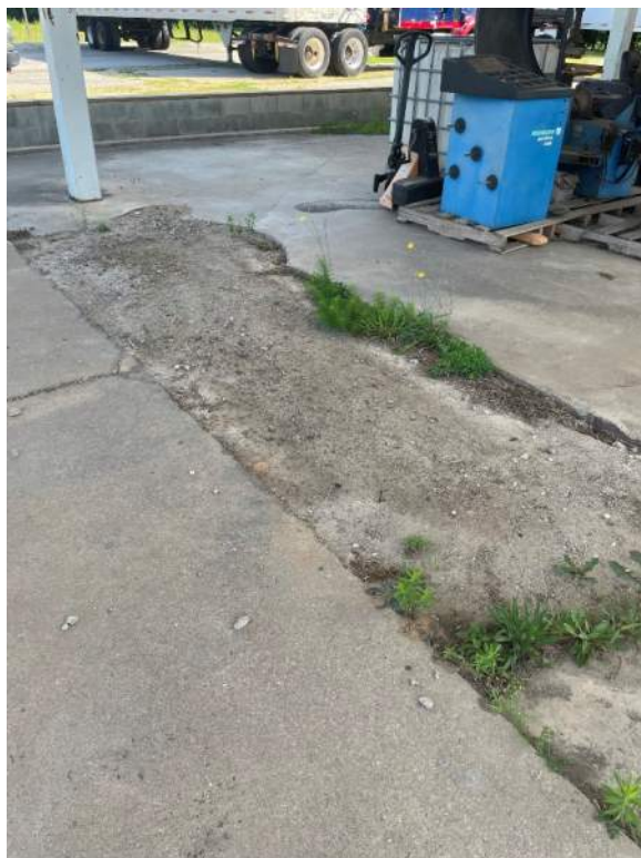
View facing west underneath the former fuel canopy.
