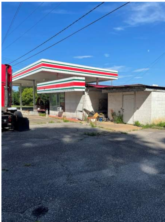
View facing west from the eastern boundary of the Project Study Area along the side of the inactive convenience store.
