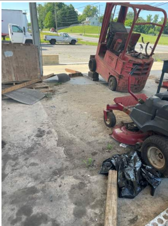
View facing west towards NC 115 displaying machinery stored underneath the former fuel canopy.
