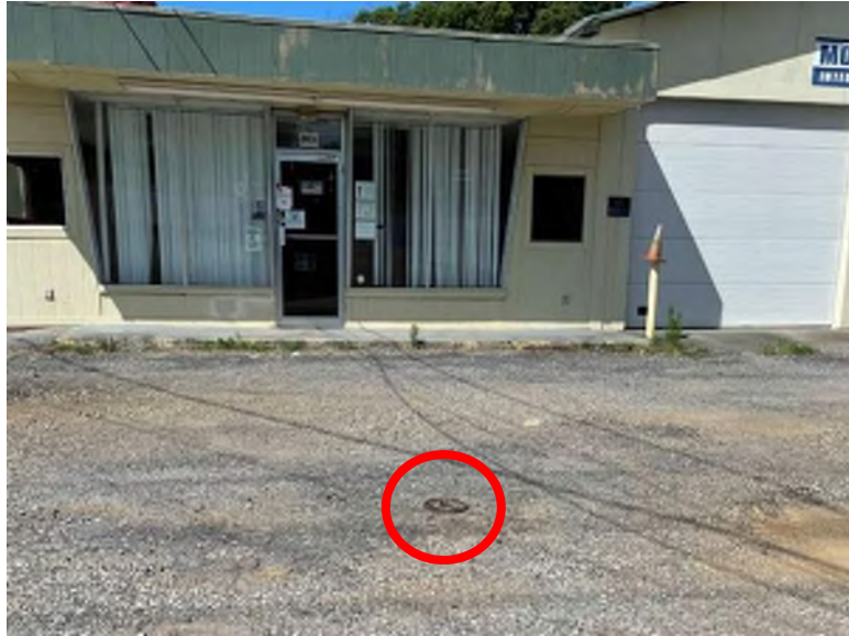
View facing west from the northeastern portion of Parcel 73 depicting an automotive store and groundwater monitoring well.
