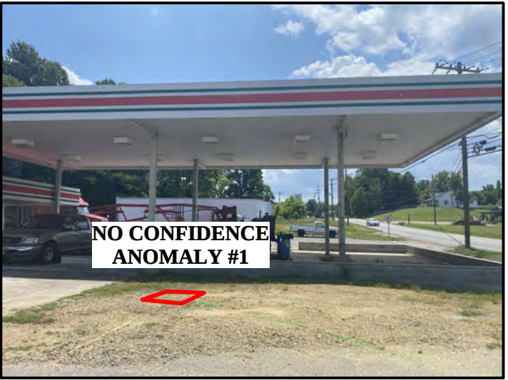
View of One No Confidence Anomaly (Facing Approximately South)
