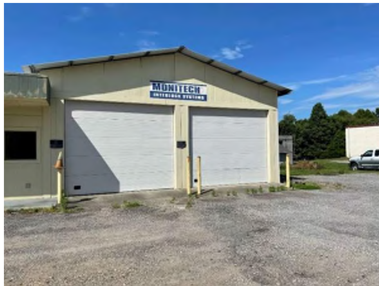
View facing west from the northeastern portion of Parcel 73, depicting an automotive garage.
