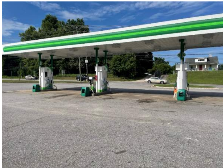
View facing west from the BP convenience store located on the eastern boundary of the parcel, towards the fuel islands and US 421.
