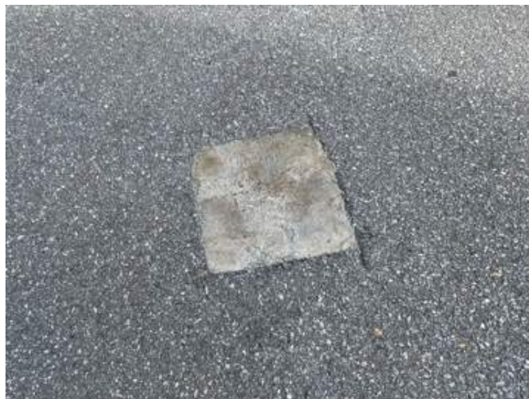
Likely closed groundwater monitoring well located in the northern area of the Project Study Area parking lot between the fuel islands and the UST bed.
