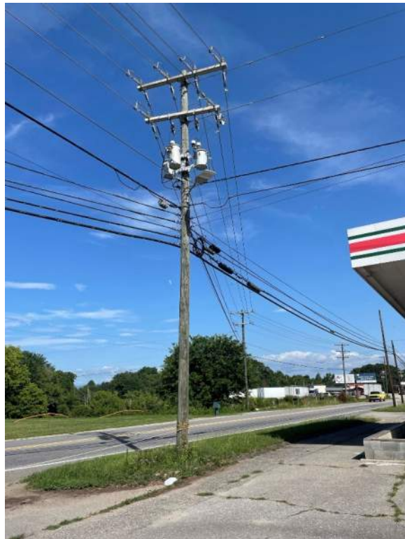
View facing north from the southwestern corner of the Project Study Area, displaying NC 115 on the western boundary of the Project Study Area and overhead power lines.
