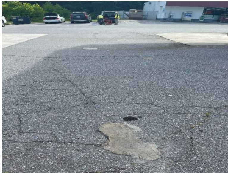
View facing east from the northwestern area of the Project Study Area between the UST bed and the fuel islands. Concrete fill purpose is unknown.
