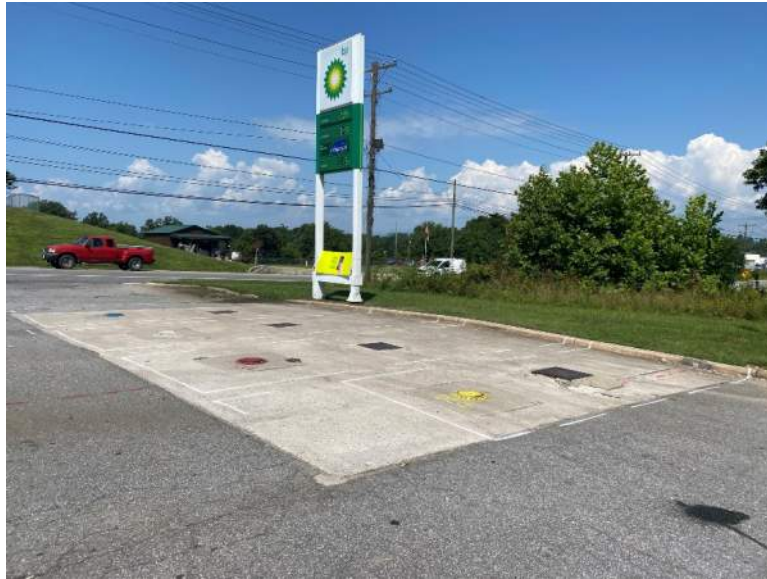
View facing northwest from the western portion of the Project Study Area, depicting four known USTs outlined with white spray paint.
