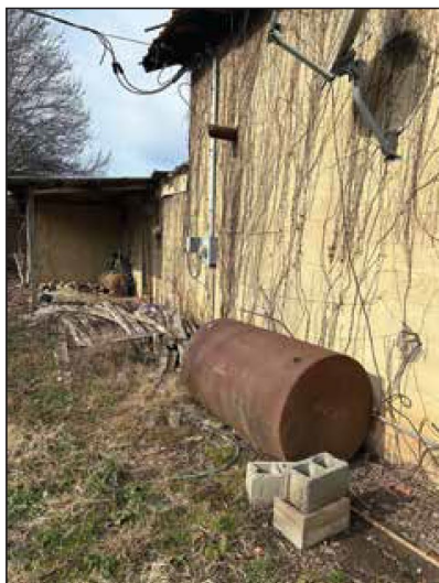
Photo 1. AST on the south side of the building (not within R/W).
