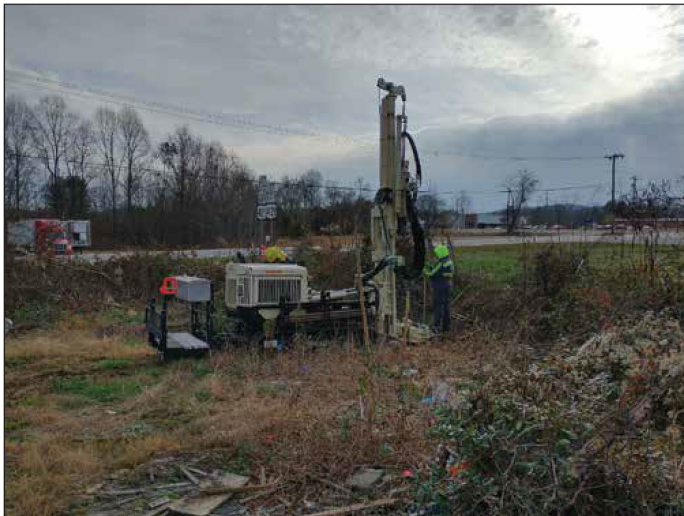
Photo 4. Carolina Soil Investigations drilling boring B-1.
