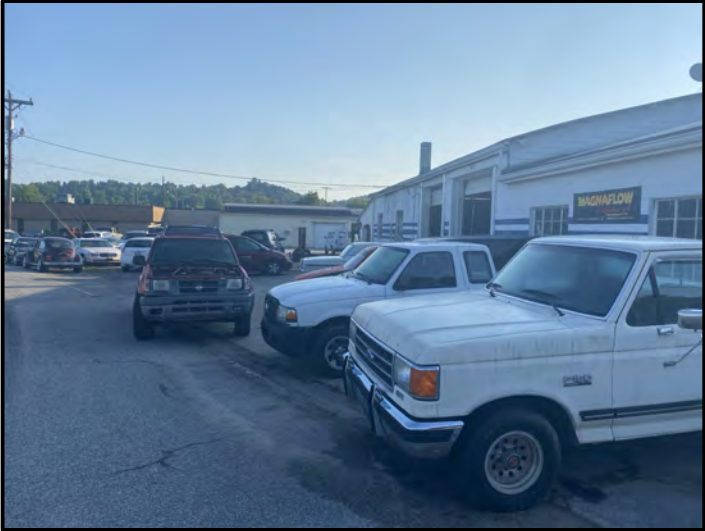
View of Survey Area (Facing Approximately North)
