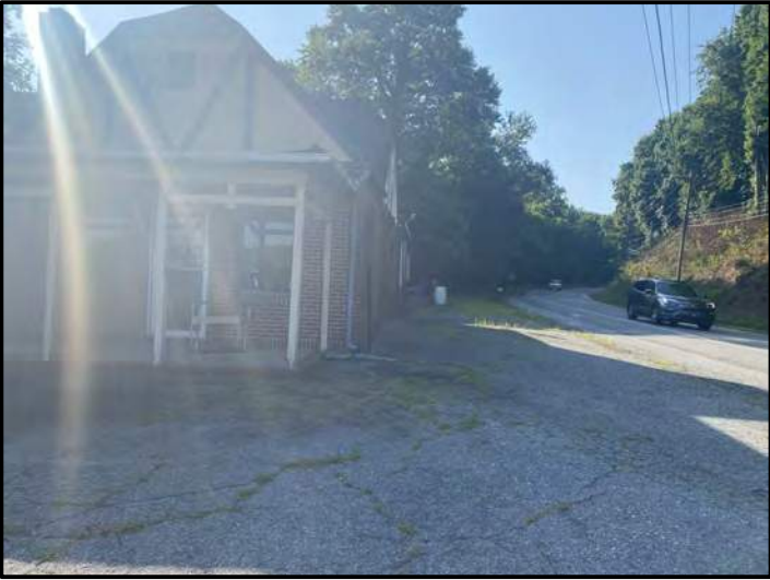
View of Survey Area (Facing Approximately Southeast)
