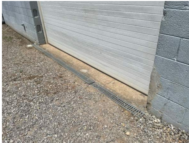
Floor drains in front of the bay door on the western side of the building facing NC 115.
