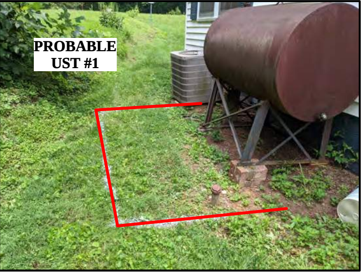
View of One Probable UST (Facing Approximately North)
