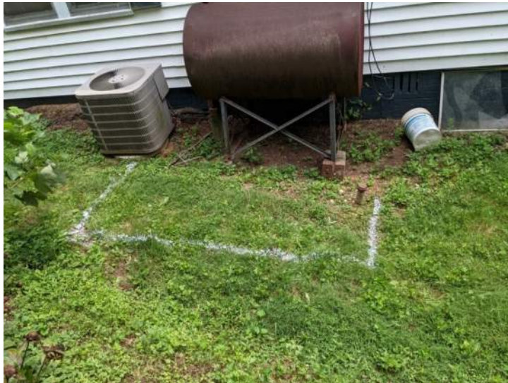
View facing east from the northwestern corner of the Project Study Area, depicting a 500-gallon AST (likely heating oil) along the northern side of the blue and white painted house in the northernmost portion of the parcel. One (1) probable heating oil UST adjacent to the AST was observed as part of the geophysical survey and was outlined with white spray paint.
