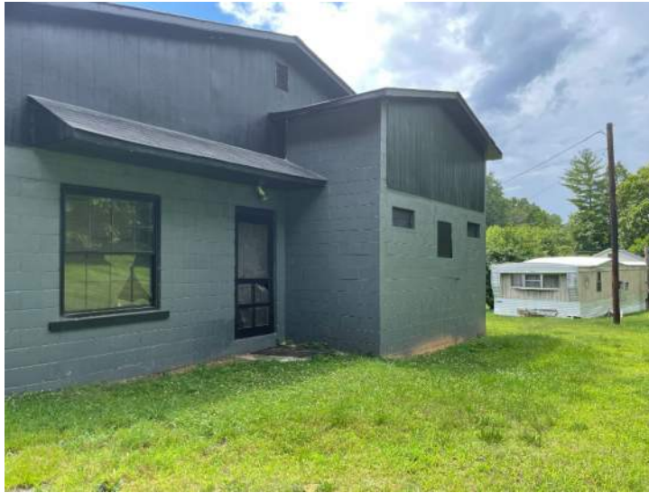
View facing west from the eastern portion of the Project Study Area, depicting the northeastern side of the gray-painted cinderblock building.
