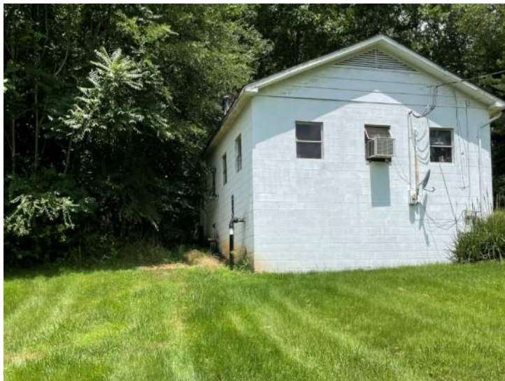
View facing northeast from the northeastern portion of the parcel, depicting the western side of the garage with two bay doors located along Cedar Lane.
