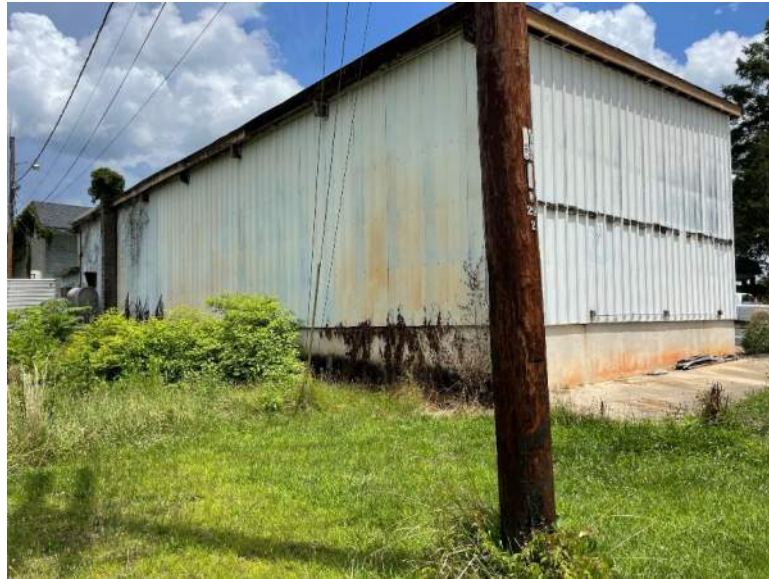
View facing east along the northern side of the automotive garage building in the central portion of the Project Study Area.
