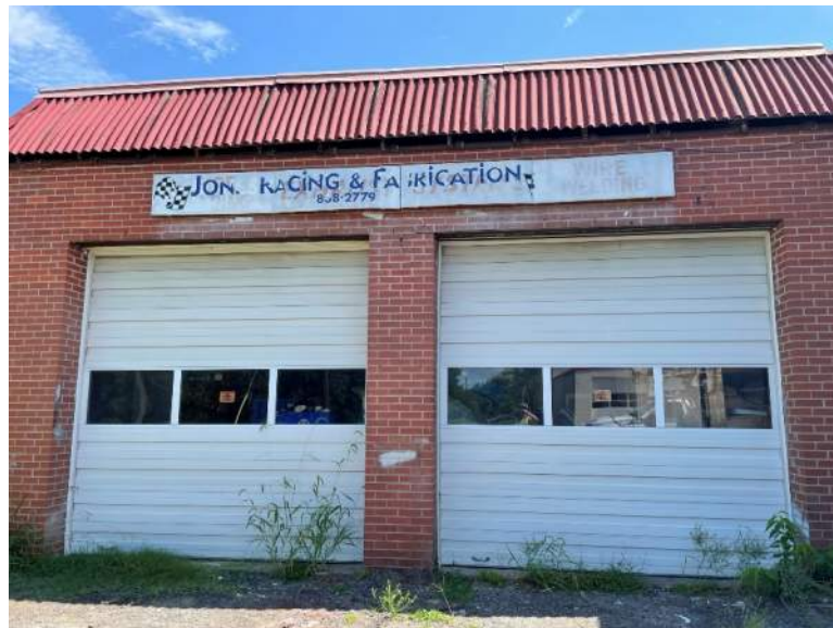
Building with two bay doors that may contain in-ground hydraulic lifts located in the northeastern portion of the Project Study Area.
