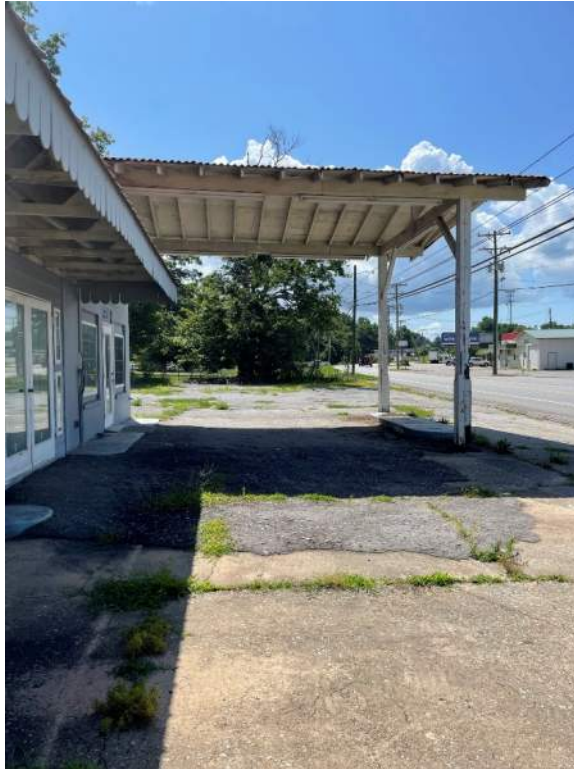
View facing southeast from the northeastern portion of the Project Study Area along NC 115.
