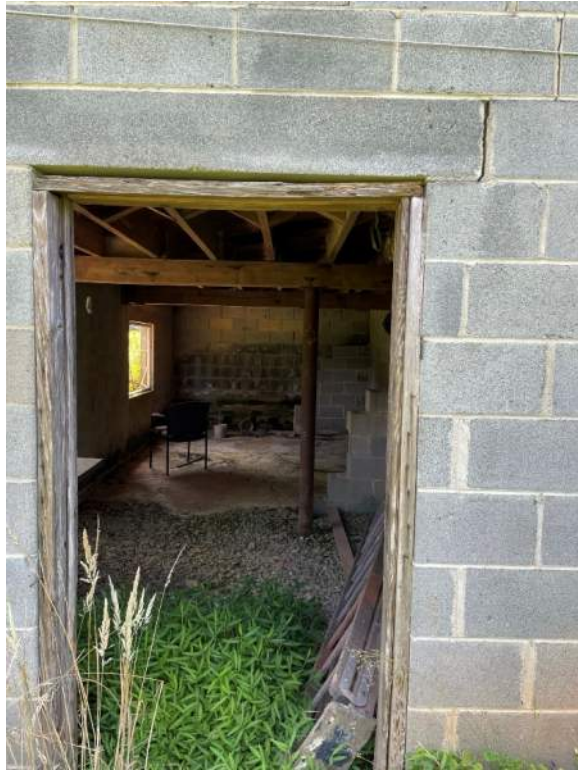
View facing into the basement entryway along the northern side of the building with two bay doors, located in the northeastern corner of the Project Study Area.
