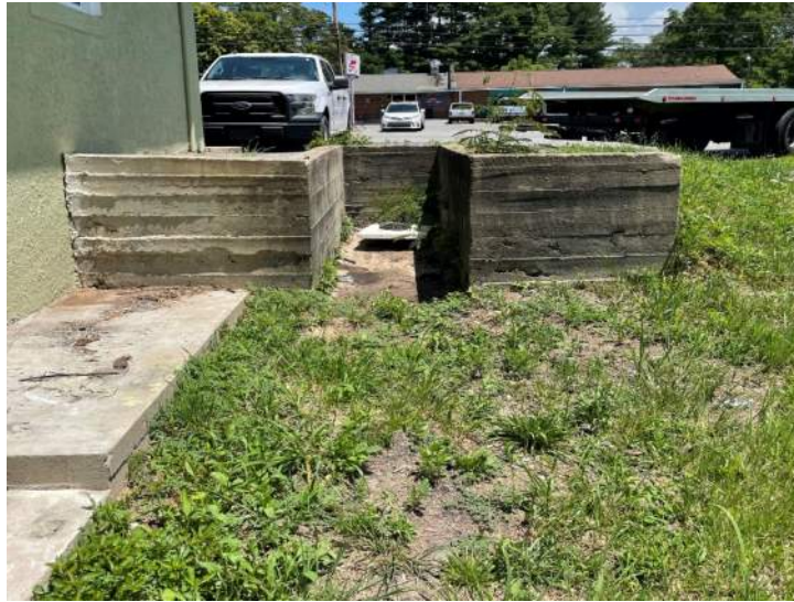
View facing northeast towards NC 115 along the southeastern side of the convenience store, depicting an earthen oil pit.
