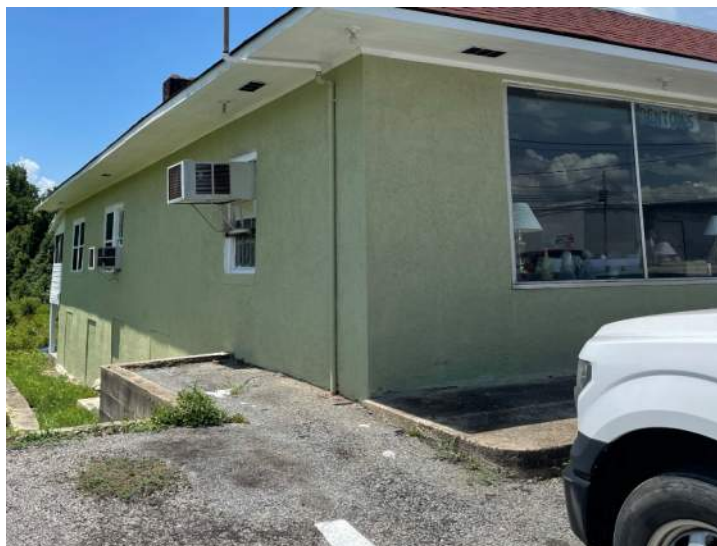
View facing west towards depicting the convenience store, the southern corner of the former UST bed, and the top of an inactive earthen oil pit.
