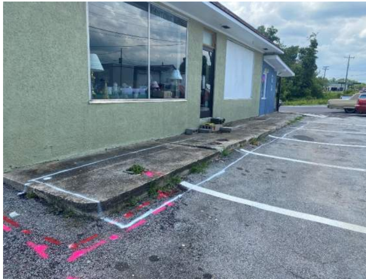
The former UST bed with three probable USTs outlined with white spray paint on the northern side of the convenience store facing NC 115.
