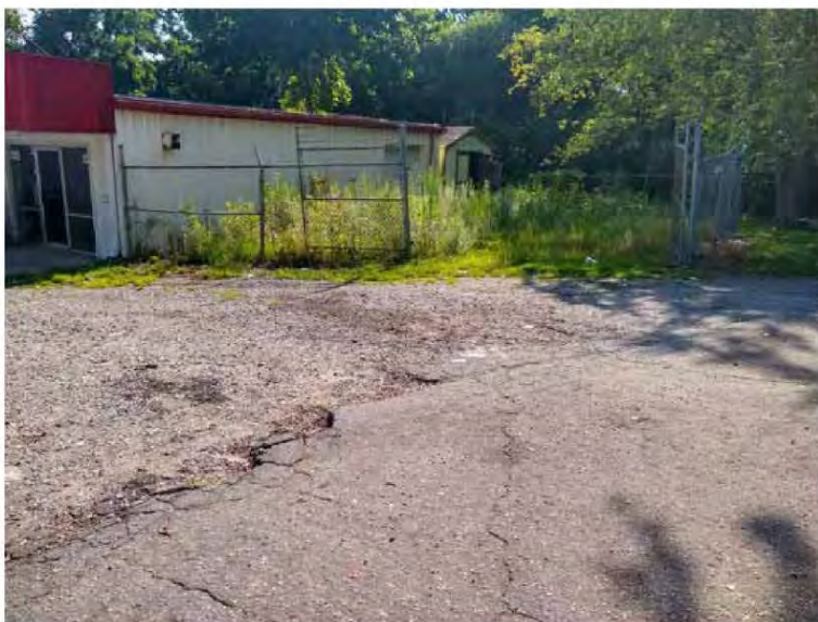
Photo 3. Possible location of former UST System on the south side of the property.
