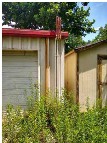
Photo 4. Vent pipes attached to the Pool & Spa building.
