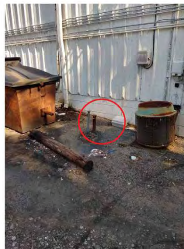
Photo 5. Additional fuel oil UST on the south side of the gas station. Tank is outside of the R/W and PUE.
