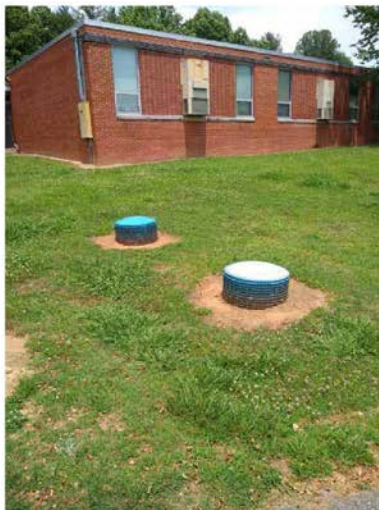
Photo 4. Risers near the southwest corner of the building likely related to a septic tank.
