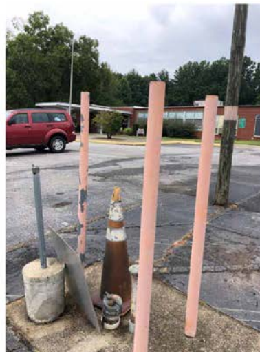
Photo 5. UST Fill and Vent pipe located in the parking lot on the south side of the school building.
