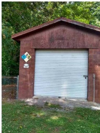
Photo 3. Storage shed west of the school building. The sign on the left side of the building indicates that the shed contains gasoline and/or diesel fuel.
