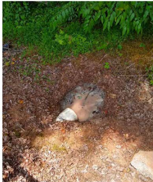
Photo 4. Example of a drain pipe located along the northern side of the property within the Temporary Construction Easement.
