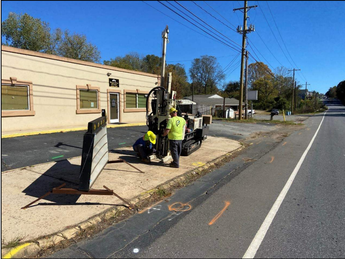
Photo 3: Geoprobe drilling boring B-4, looking northeast.
