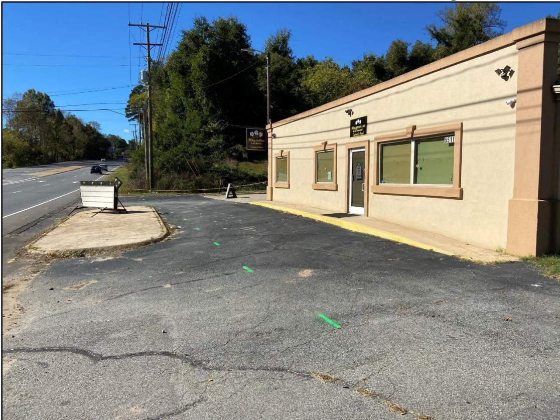
Photo 8: Final conditions of the site after field work, looking west.
