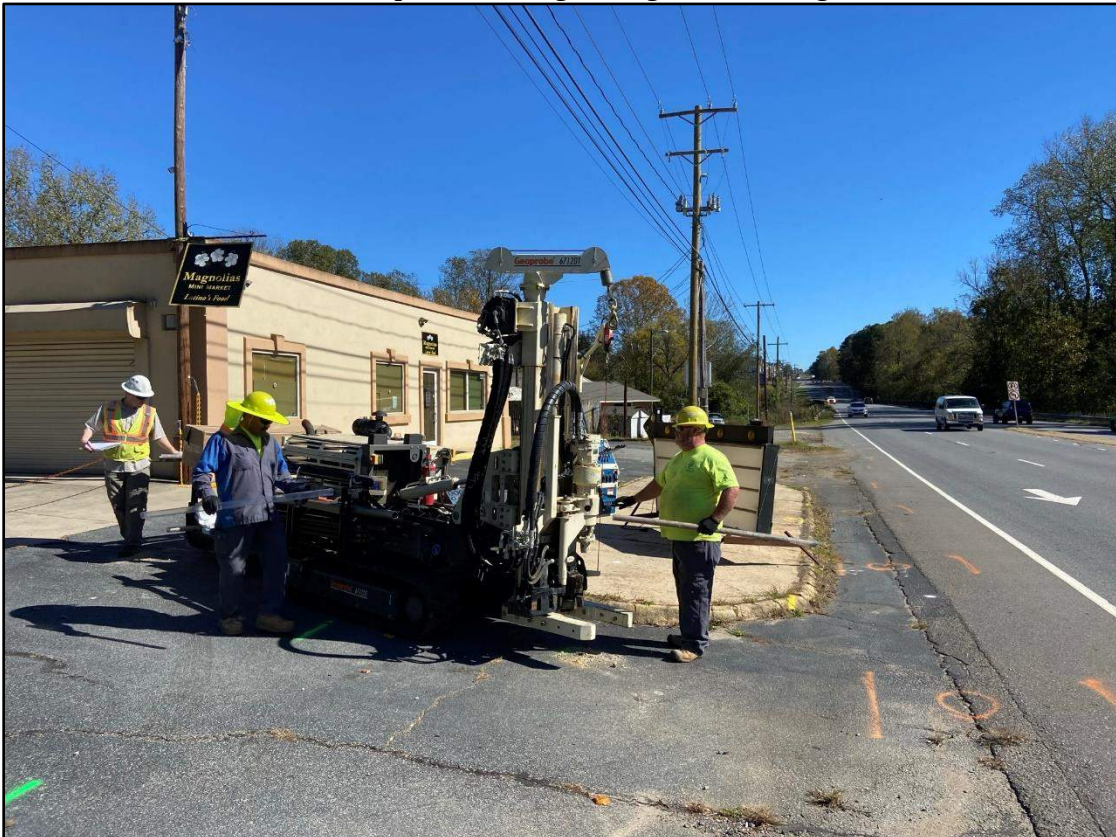
Photo 4: Geoprobe drilling boring B-3, looking east.
