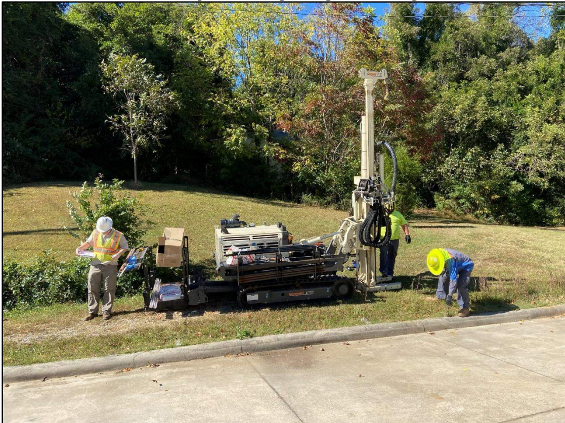
Photo 6: Geoprobe drilling boring B-1, looking west.
