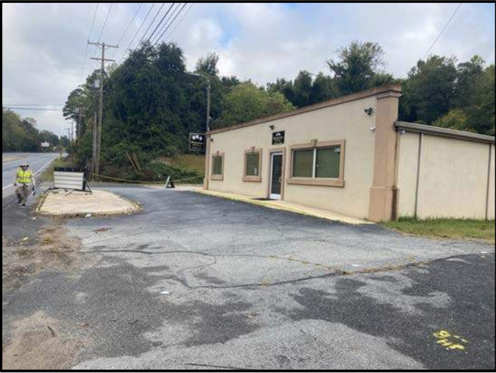
View of Survey Area (Facing Approximately West)
