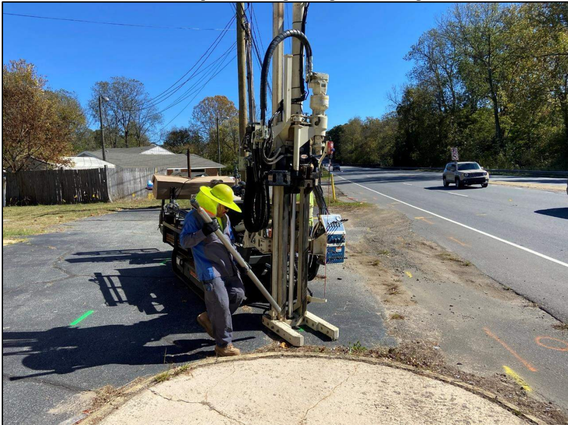
Photo 2: Geoprobe drilling boring B-5, looking east.
