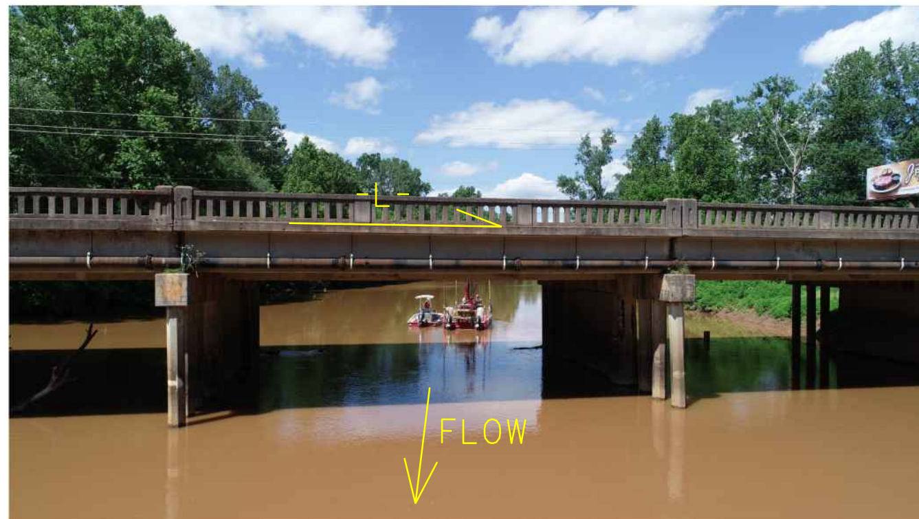
Photo #2: Existing Bridge 82 on US 29 /74 over South Fork Catawba River looking upstream
