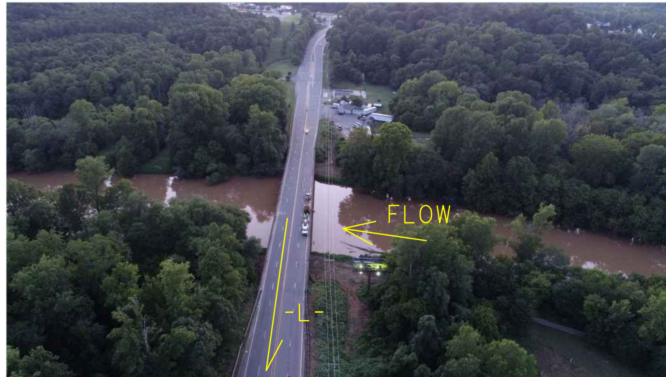
Photo #1: Existing Bridge 82 on US 29 /74 over South Fork Catawba River looking west (downstation)
