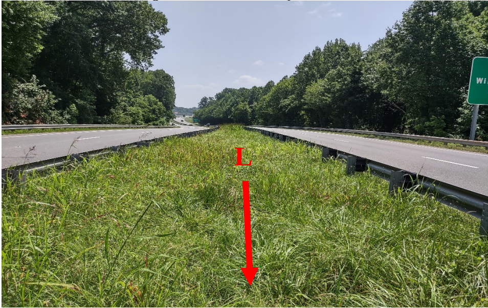
Looking Downstation from Upstation of EB2
