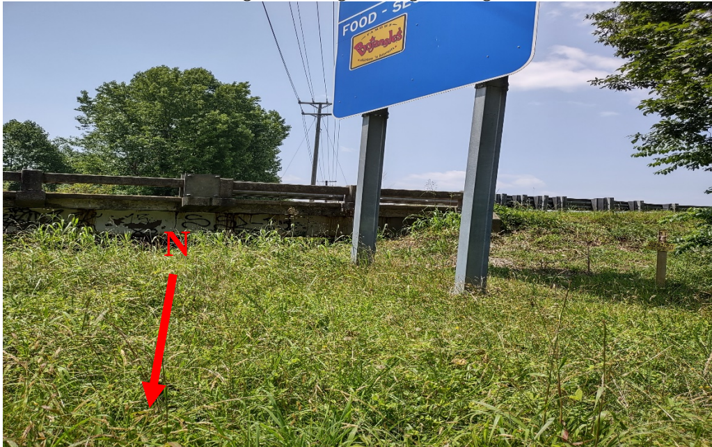
Looking Left to Right Along Existing EB1
