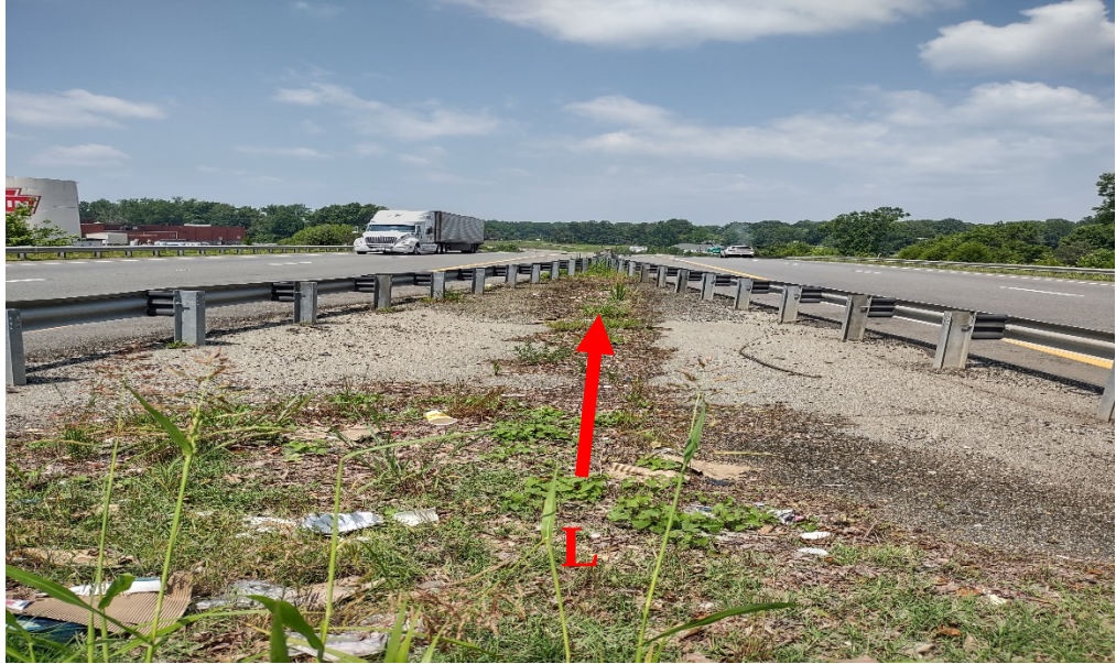
Looking Upstation From Downstation of End Bent-1
