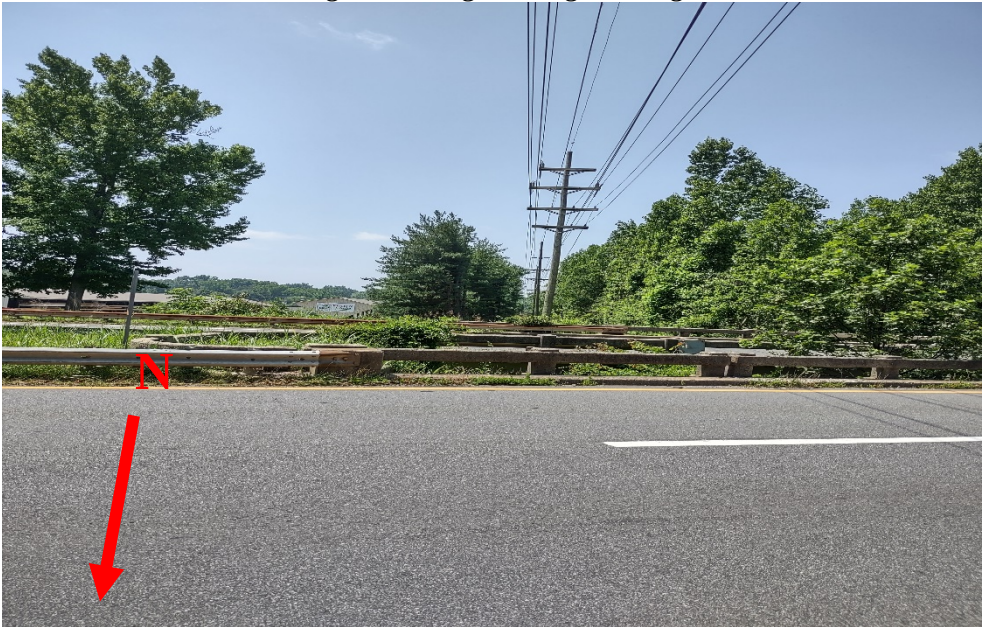
Looking Left to Right Along Existing EB2
