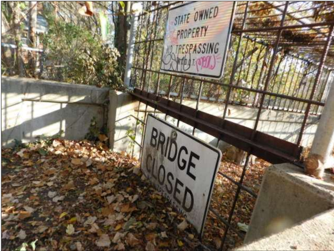
LOOKING SOUTH (BRIDGE CLOSED, REBAR WELDED ACROSS APPROACH TO PREVENT PEDESTRAIN ENTRANCE TO STRUCTURE)
