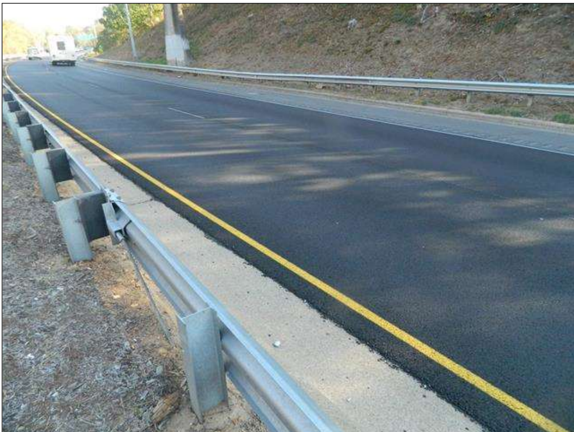
NEW WEARING SURFACE UNDER STRUCTURE
