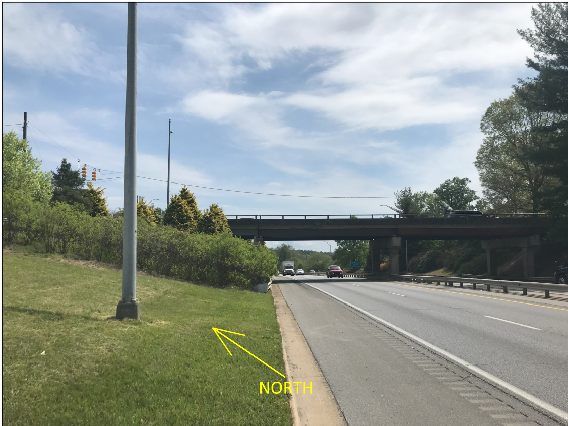
PHOTO 4: VIEW FROM PROPOSED BRIDGE 242 ALONG I-26/I-240 (-L-), FACING UPSTATION
