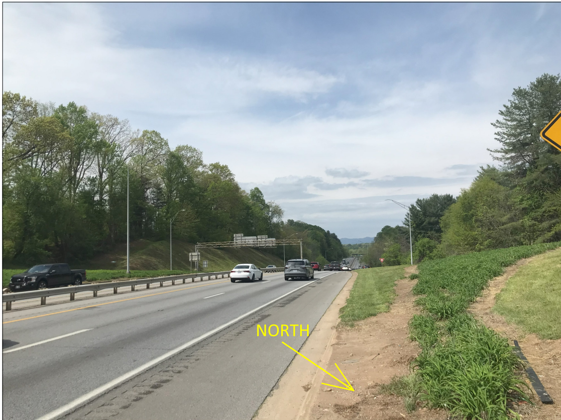
PHOTO 3: VIEW FROM PROPOSED BRIDGE 242 ALONG I-26/I-240 (-L-), FACING DOWNSTATION
