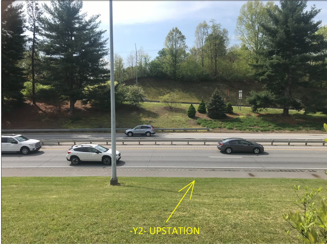
PHOTO 2: VIEW FROM PROPOSED BRIDGE 242 AT END BENT 1, FACING SOUTH-SOUTHWEST
