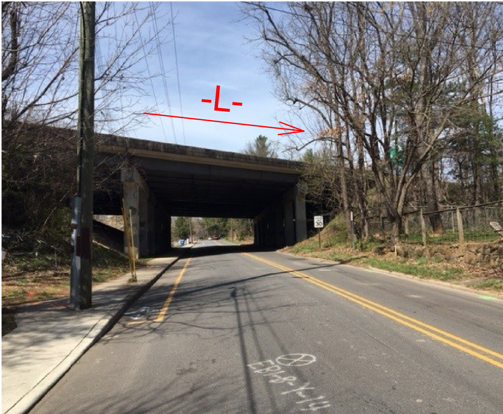
ON STATE STREET ALONG -Y14- ALIGNMENT LOOKING NORTH
