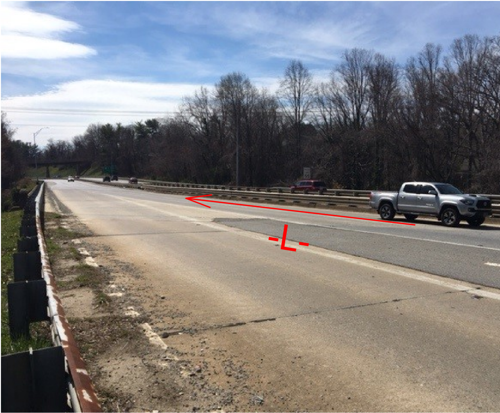
END BENT 1 LOOKING EAST
