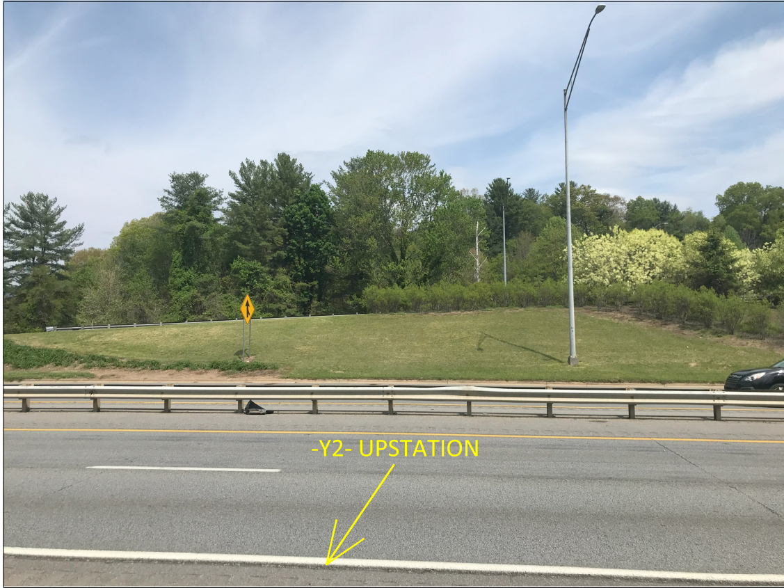
PHOTO 1: VIEW FROM PROPOSED BRIDGE 242 AT END BENT 2, FACING NORTH-NORTHEAST
