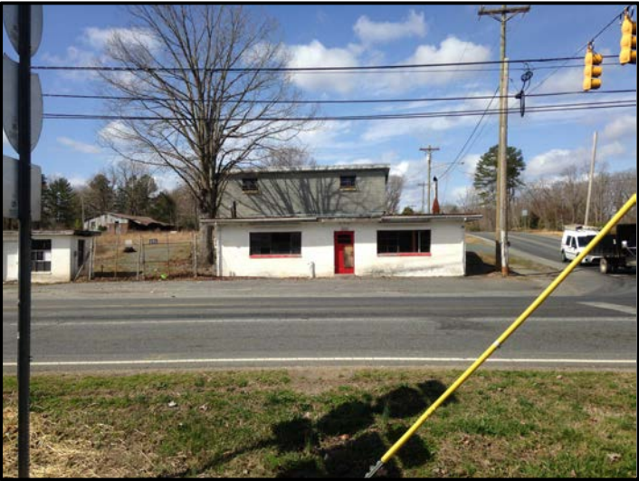
View of Survey Area (Facing Approximately West)
