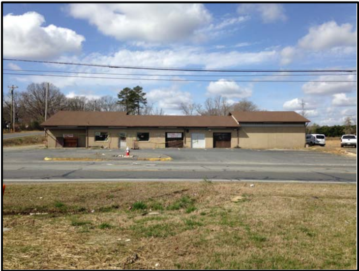
View of Survey Area (Facing Approximately West)
