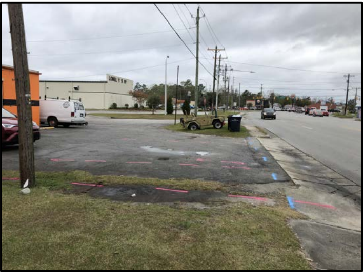
View of Survey Area (Facing Approximately West)
