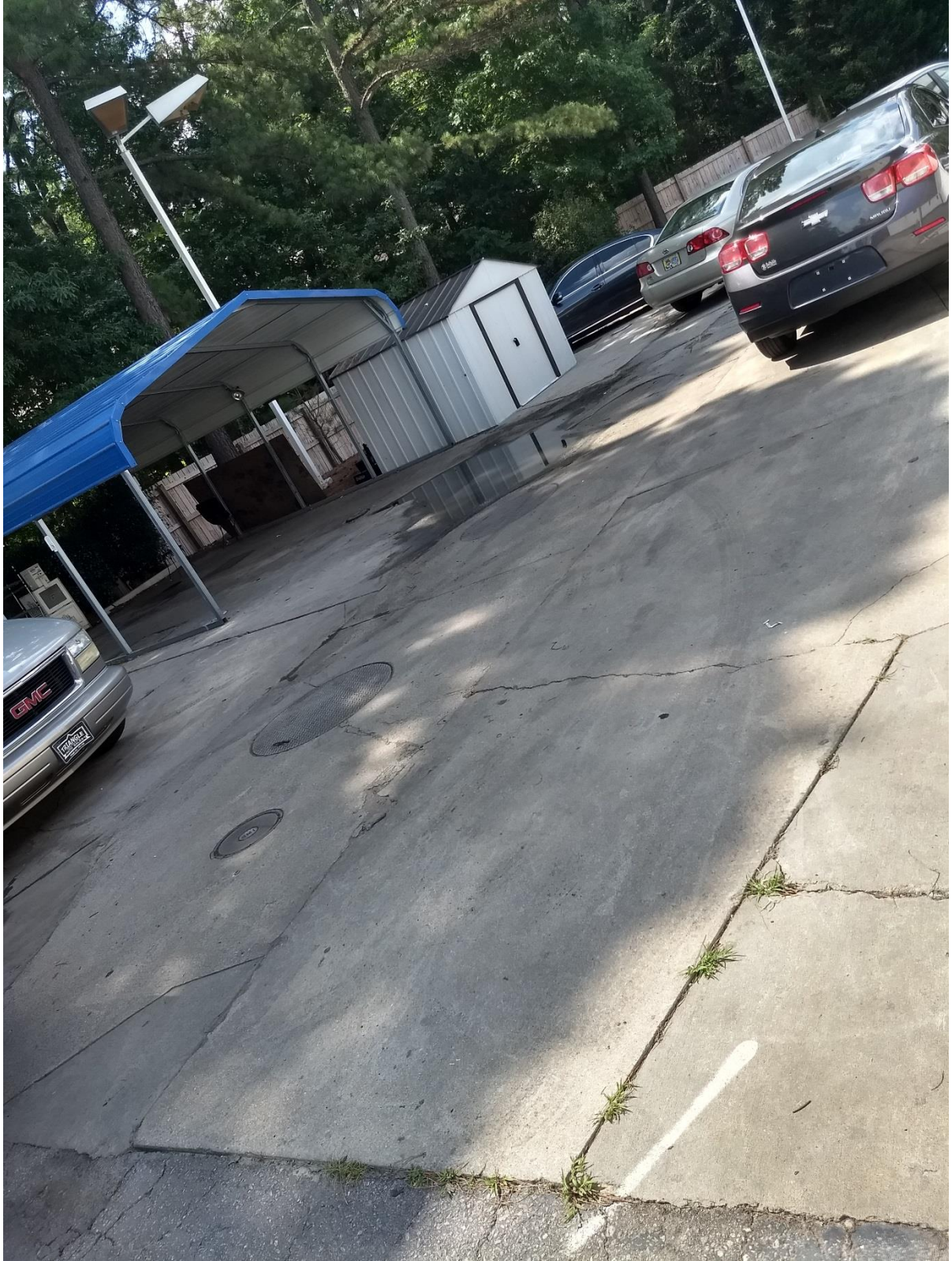
USTs behind the main building.
