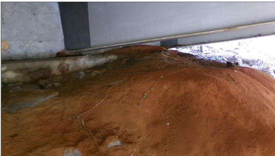
SOIL BUILD UP AT END BENT 2 UNDER BAYS 2 AND 3
