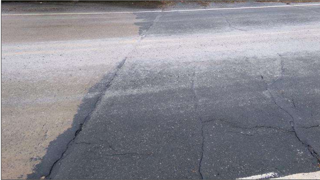
SOUTH APPROACH ASPHALT WEARING SURFACE 3/8 INCH WIDE CRACKS
