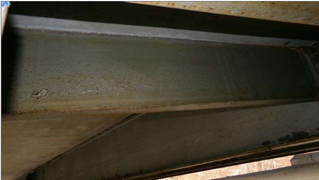
TYPICAL END DIAPHRAGM AT BENT 1
