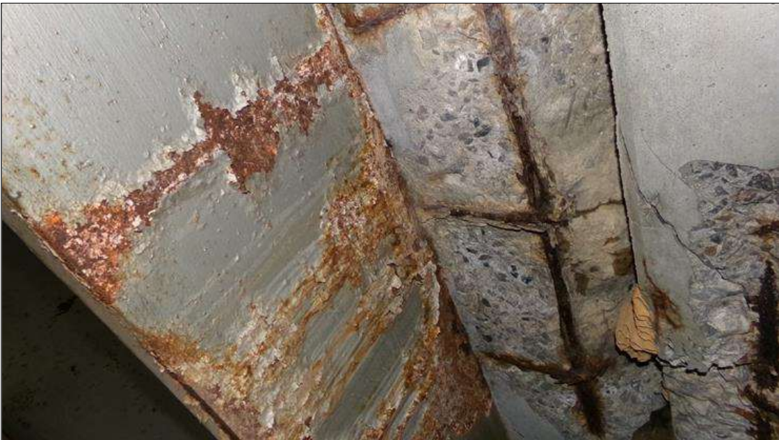
Span 2 Deck: SPALL (4FEET X 12INCHES X 2INCHES SPALL) WITH EXPOSED SCALING TO REBAR TO BOTTOM OF DECK IN BAY 2 OVER BENT 1. UP TO 90 PERCENT SECTION REMAINING IN THE EXPOSED REBAR. (PAR)
