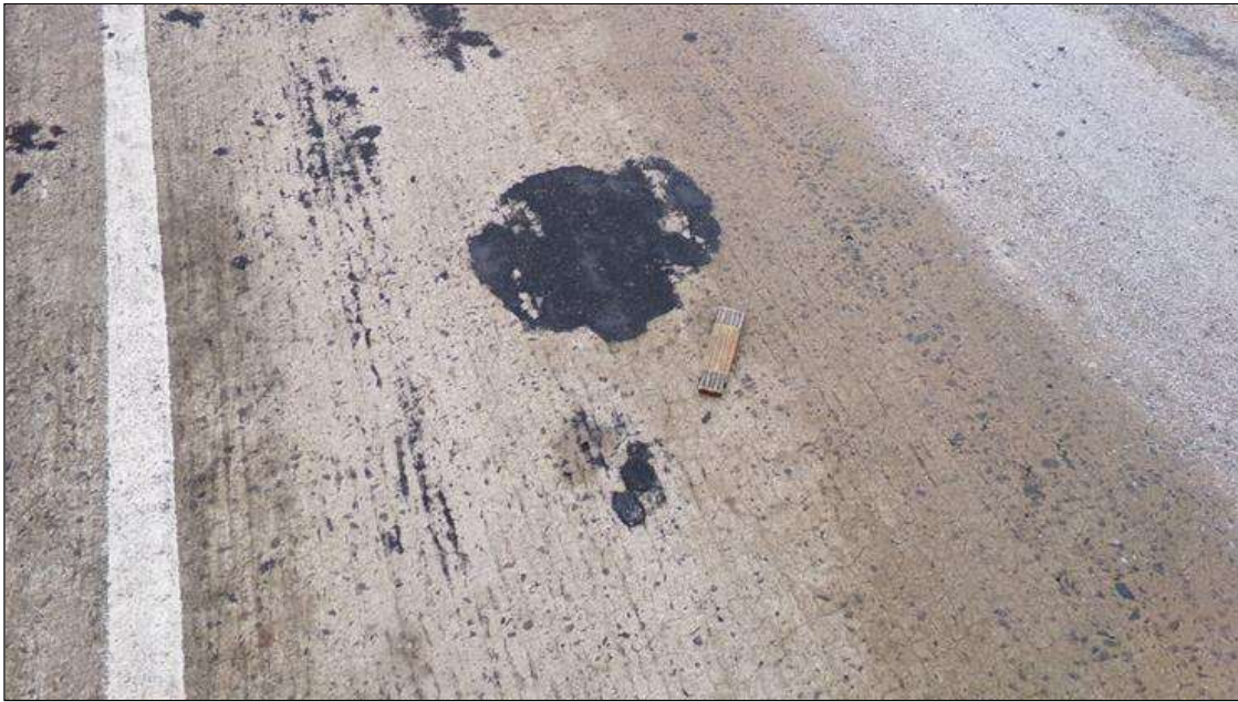
Span 1 Deck: SOUND PATCH (16INCHES DIAMETER) IN RIGHT LANE, 6FEET FROM NEAR END (SIMILAR IN LEFT LANE AT MID SPAN)
