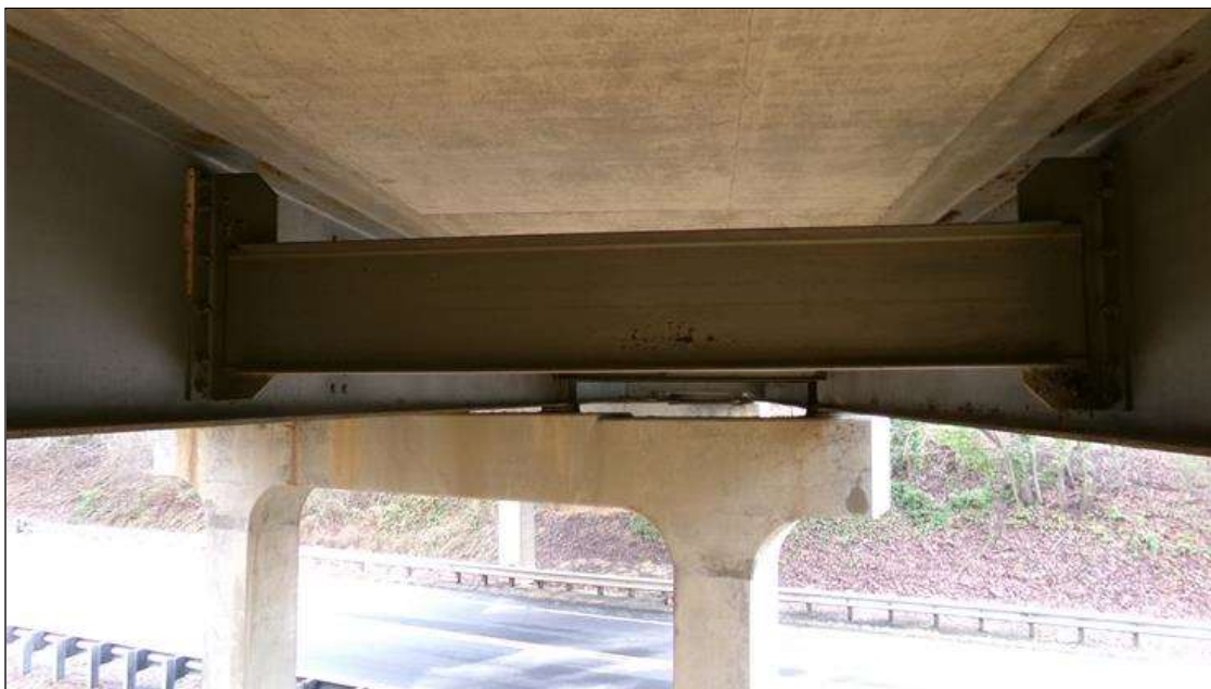
TYPICAL INTERMEDIATE DIAPHRAGM IN SPAN 3
