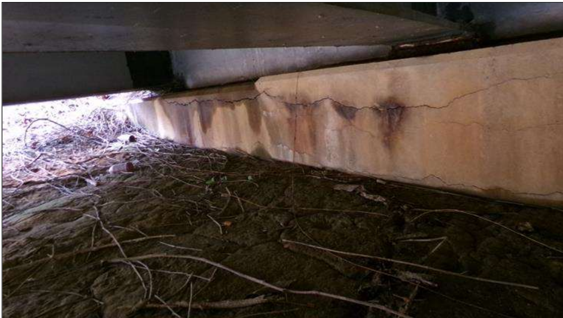
End Bent 1 Cap 1: HORIZONTAL OPEN CRACKING (HAIRLINE TO 1/8 INCH) WITH RUST STAINING THRU OUT FACE OF CAP
