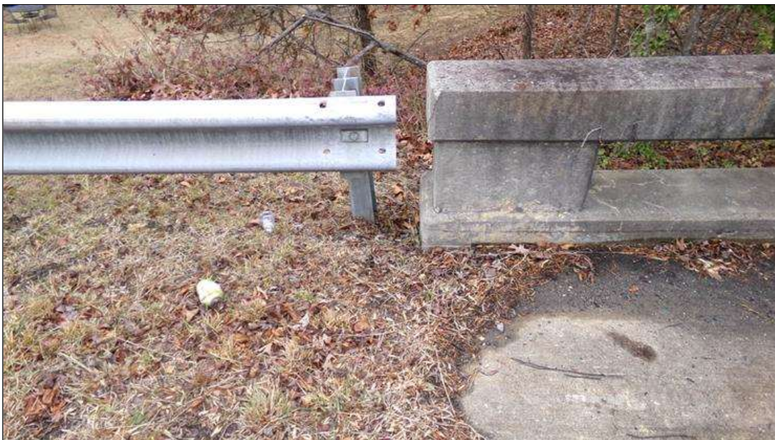
GUARDRAIL DOES NOT ATTACH TO RAIL AT SOUTHWEST CORNER
