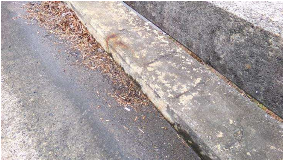
Span 1 Right Bridge Rail: 9 SHALLOW SPALL (UP TO 10INCHES X 3INCHES X 1/4INCH) WITH EXPOSED REBAR TO TOP OF CURB THRU OUT, MOSTLY AT NEAR END. NO MEASUREABLE SECTION LOSS IN THE EXPOSED REBAR.
