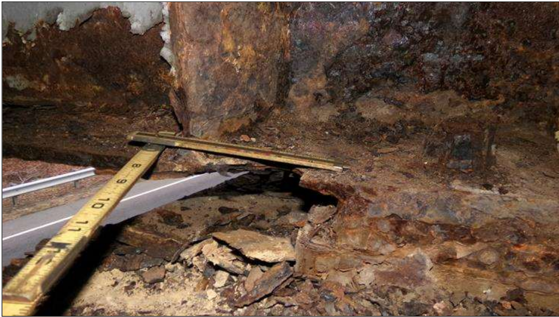
Span 2 Beam 4: BOTTOM FLANGE SECTION LOSS (UP TO 100 PERCENT) FOR 1 INCH DIAMETER. 3/8 (50PERCENT) AVERAGE REMAINING FOR FULL WIDTH FOR 16INCHES AT NEAR END (PAR)
