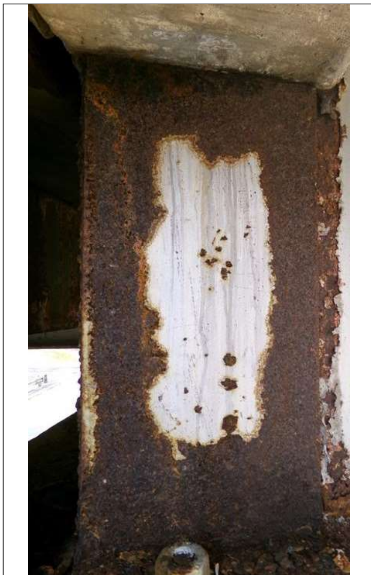
Span 3 Beam 4: WEB PLATE REPAIR (1FOOT X FULL HEIGHT X 1/2INCH THICK) TO NEAR END
