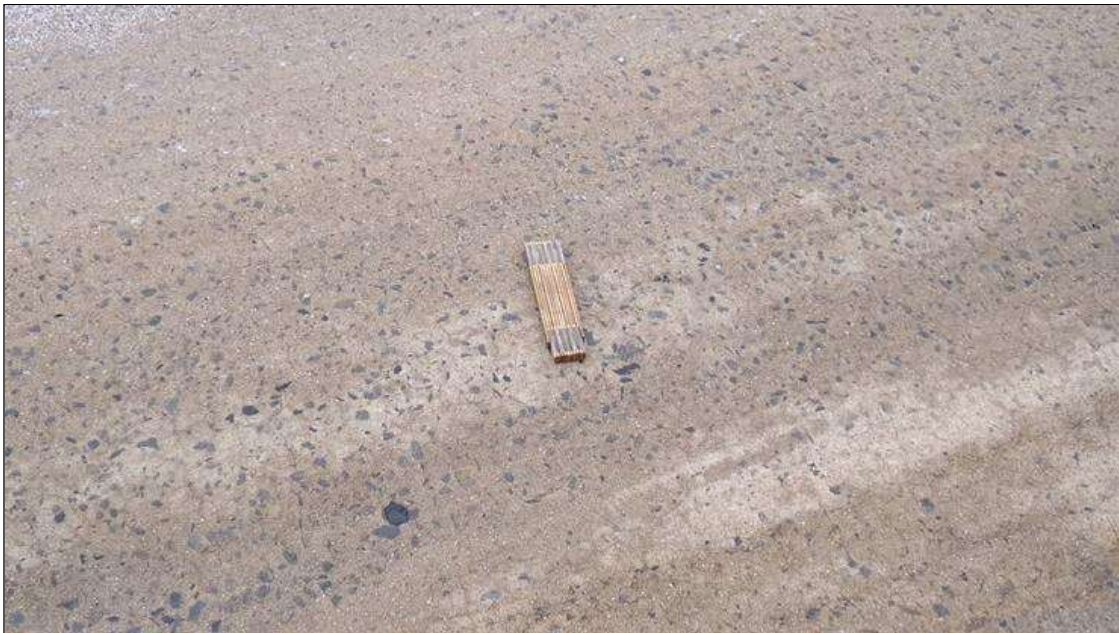
Span 3 Deck: MAP CRACKING (UP TO 1/16INCH) THRU OUT DECK.
