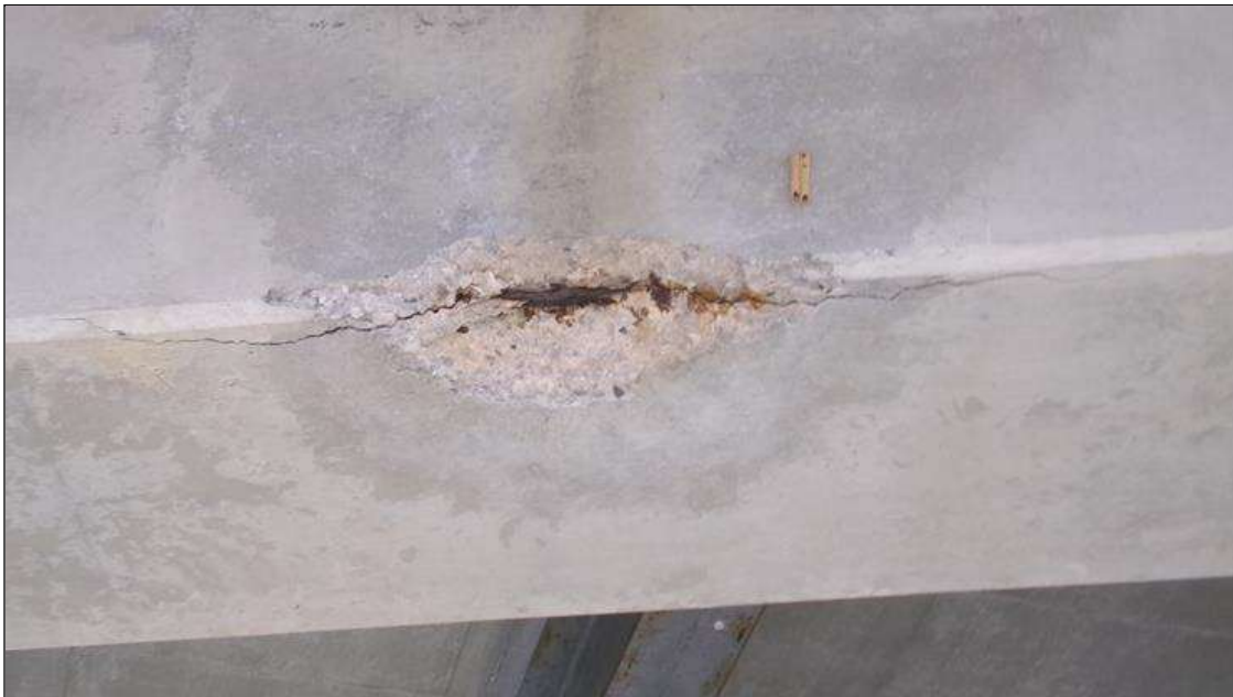
Bent 1 Cap 1: SPALL (2.5FEET X 1FOOT X 6INCHES) WITH EXPOSED SCALING REBAR TO FAR BOTTOM CORNER OF CAP UNDER BAY 2. UP TO 60 PERCENT REMAINING IN THE EXPOSED REBAR. (PAR)
