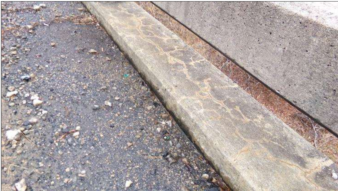
Span 3 Right Bridge Rail: INTERMITTENT TRANSVERSE CRACKING (LESS THAN 1/16INCH) AND WEATHERING WITH EXPOSED AGGREGATE AND MINOR EFFLORESCENCE THRU OUT RAIL.
