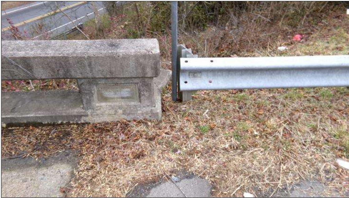
GUARDRAIL DOES NOT ATTACH TO RAIL AT SOUTHEAST CORNER
