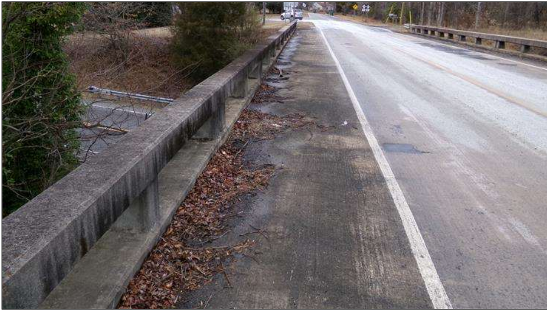
Span 2 Deck: 110 SQUARE FEET ASPHALT PATCHES THRU OUT RIGHT LANE WITH SPALLING AT PATCH PERIMETERS
