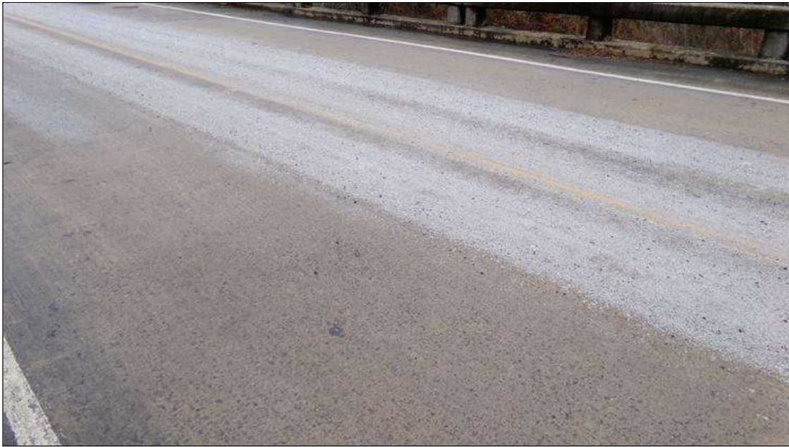
SPAN 1 TOP OF DECK (SALT BRINE ON TOP OF DECK) SPANS 2 AND 3 TYPICAL
