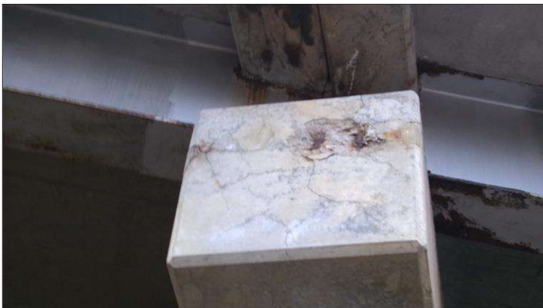
Span 2 Deck: SPALL (1FOOT X 10INCH X 1INCH) WITH EXPOSED SCALING REBAR TO RIGHT OVERHANG AT NEAR END. UP TO 90 PRECENT SECTION REMAINING IN THE EXPOSED REBAR (PAR)
