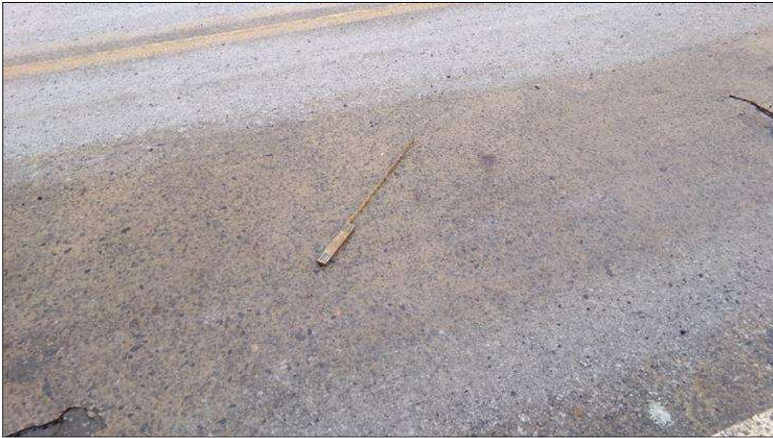
Span 2 Deck: WEAR WITH EXPOSED AGGREGATE THRU OUT DECK
