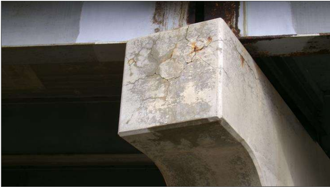
Bent 2 Cap 1: OPEN MAP CRACKING (UP TO 1/8 INCH) TO LEFT FACE OF CAP AND VERTICAL AND HORIZONTAL OPEN CRACKING (UP TO 1/8 INCH) TO RIGHT FACE AND RIGHT SIDE OVERHANG. HAS ACTIVE LEAKAGE ON FACE OF CAP AT TIME OF INSPECTION
