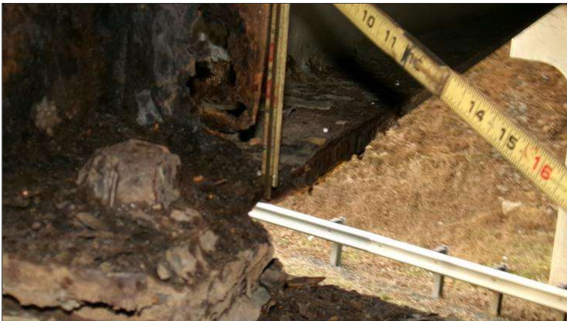
Span 2 Beam 1: BOTTOM FLANGE SECTION LOSS (3/8INCH REMAINS) FULL WIDTH FOR 16INCHES AT NEAR END. WEB STIFFENER (UP TO 100 PERCENT SECTION LOSS) 4INCHES X 4INCHES (PAR)
