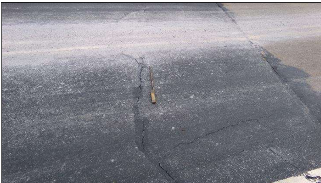
NORTH APPROACH ASPHALT WEARING SURFACE 3/8 INCH WIDE CRACKS
