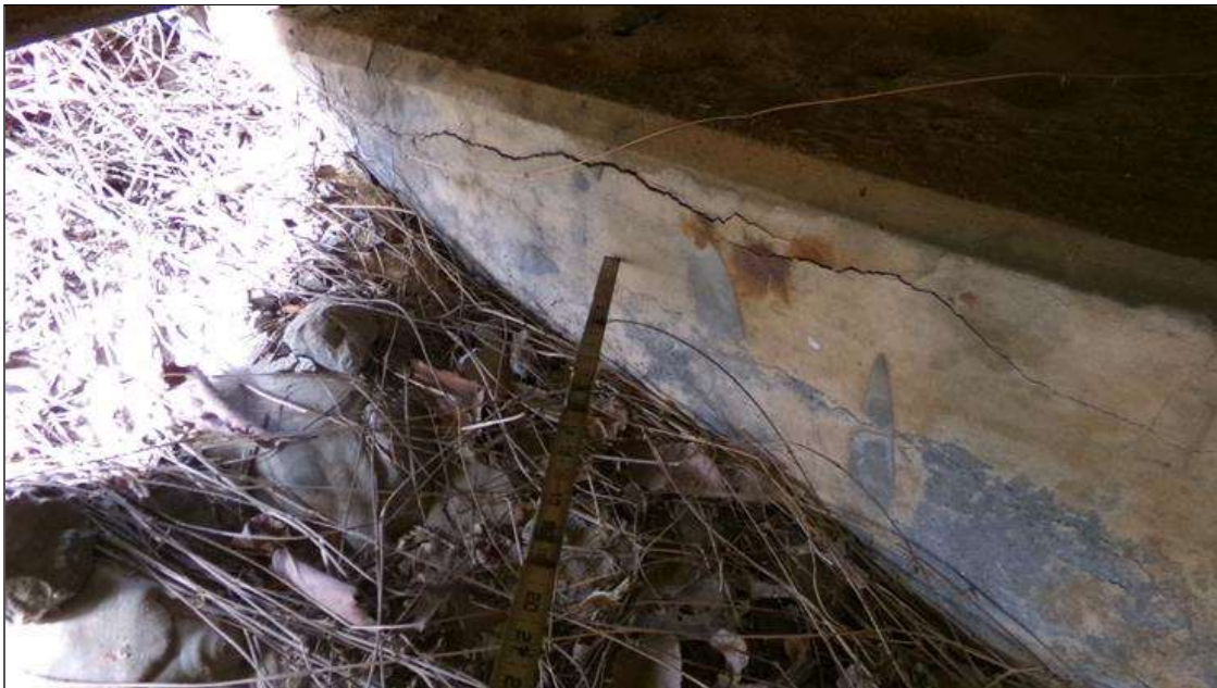
End Bent 2 Cap 1: HORIZONTAL OPEN CRACKING (HAIRLINE TO 1/8INCH) WITH RUST STAINING THRU OUT FACE OF CAP
