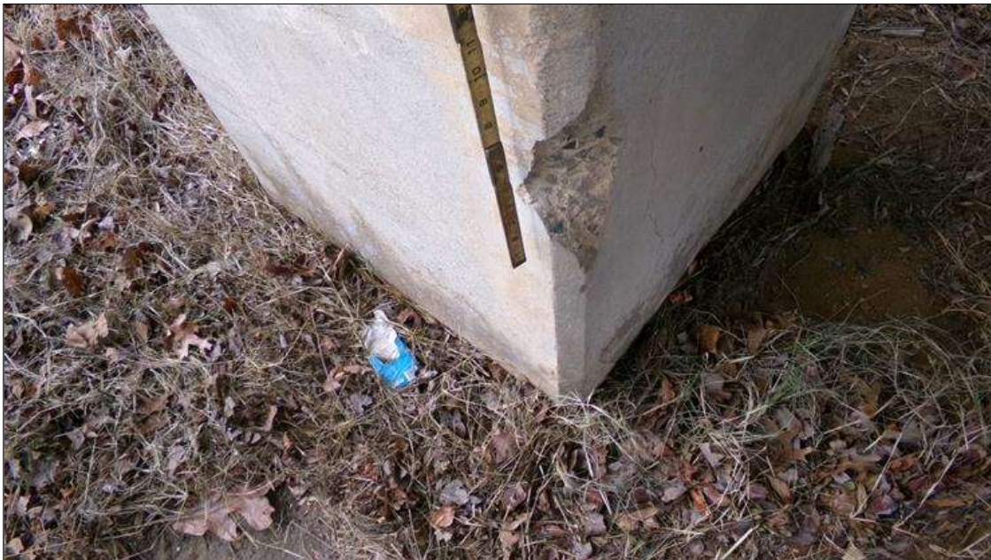
Bent 2 Pile 1: SPALL (9INCHES X 3INCHES X 2INCHES DEEP) TO NEAR RIGHT CORNER AT BASE
