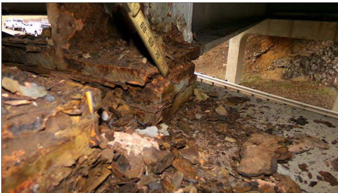
Span 1 Beam 2 - Far Bearing: SURFACE SCALING TO BEARING
