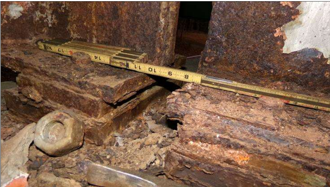
Span 3 Near Bearing: SPAN 3 BEAM 4 NEAR BEARING ANCHOR BOLT NUT BROKEN AND MISSING (PAR)
