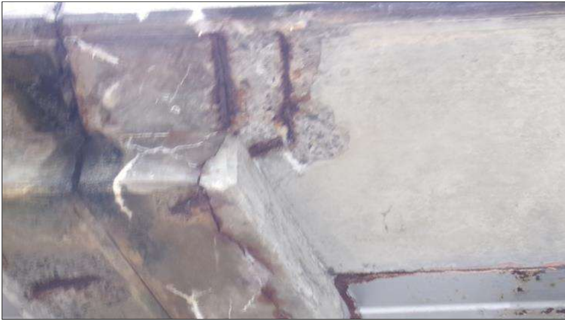
Span 2 Deck: SPALL (20INCHES X 1FOOT X 1INCH) WITH EXPOSED SCALING REBAR AND TRANSVERSE OPEN CRACKING AT LEFT SIDE OVERHANG AT FAR END. UP TO 90 PERCENT REMAINING IN THE EXPOSED REBAR (PAR)
