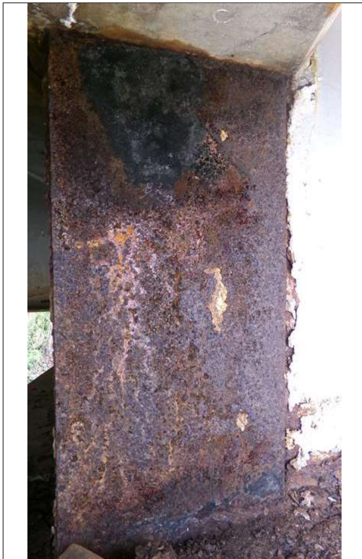
Span 2 Beam 4: WEB PLATE REPAIR (1FOOT X FULL HEIGHT X 1/2INCH THICK) AT NEAR END
