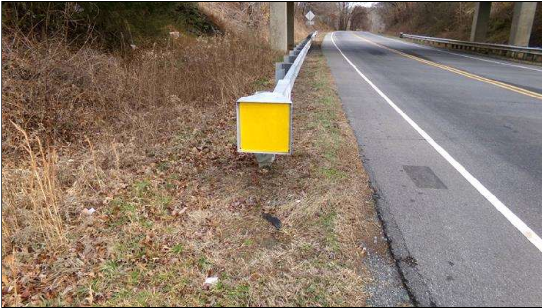
GUARDRAIL END TERMINAL FOR WEST BOUND LANE UNDERNEATH BRIDGE REPAIRED SINCE LAST INSPECTION (2024 INSPECTION)
