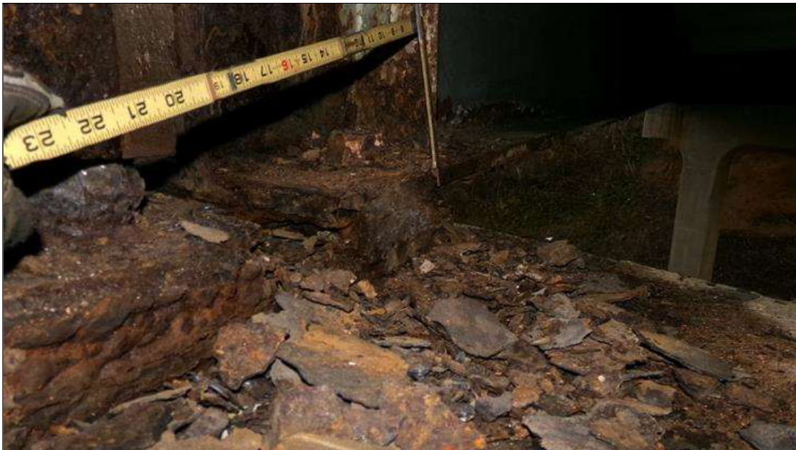
Span 2 Beam 4: BOTTOM FLANGE SECTION LOSS (21 PERCENT SECTION LOSS, 3/16 INCH SECTION LOSS, 11/16 INCH REMAINS) FULL WIDTH FOR 16 INCHES AT FAR END. SECTION LOSS UP TO 1/16 INCH (3/16 INCH REMAINS) ON THE LEFT STIFFENER FOR 2 INCHES HIGH AT BOTTOM. (PAR)
