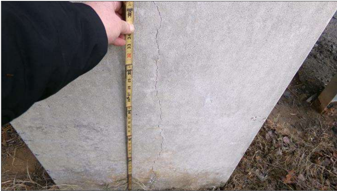
Bent 2 Pile 1: FULL HEIGHT VERTICAL CRACKING (HAIRLINE TO 1/16INCH) THRU OUT ALL FACES OF COLUMN
