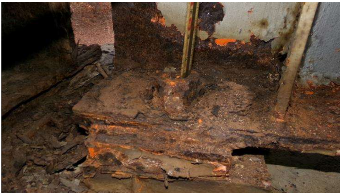
Span 1 Near Bearing: LEFT ANCHOR BOLT IS SHORT AND NOT FULLY THREADED
