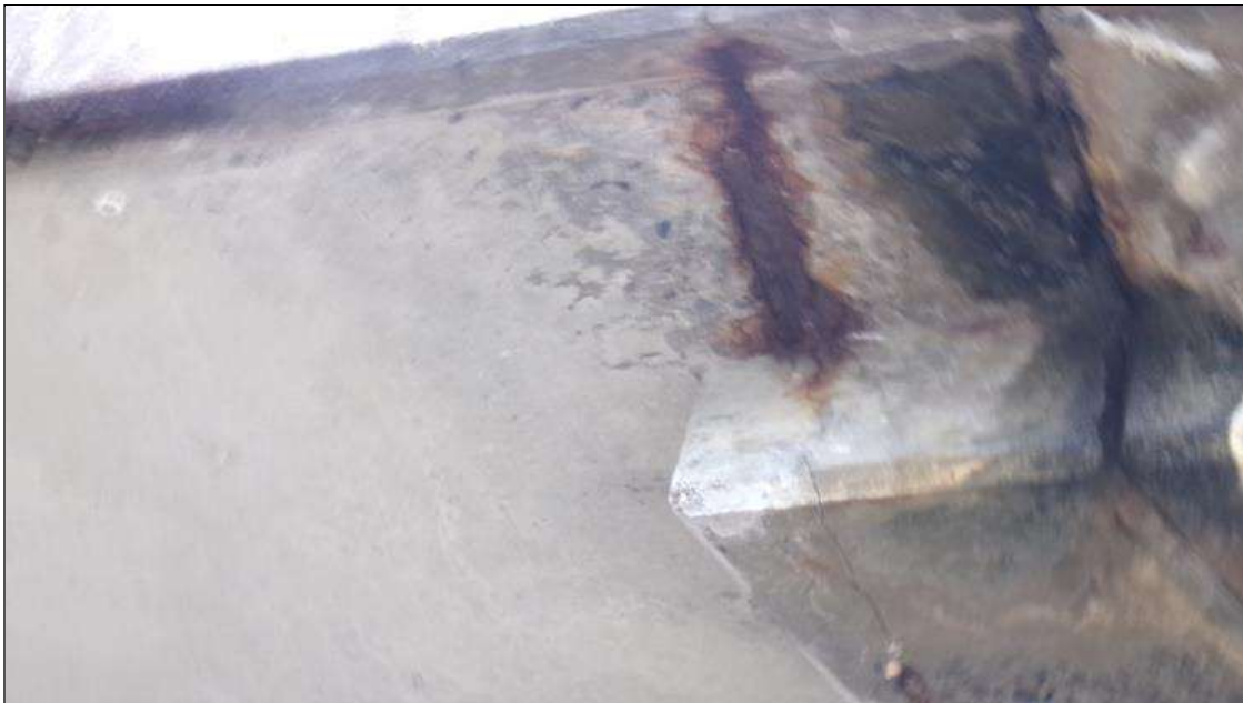
Span 3 Deck: 2 SPALLS (16INCHES X 1FOOT X 1INCH) WITH EXPOSED SCALING REBAR TO LEFT SIDE OVERHANG AT NEAR END. UP TO 90 PERCENT REMANING IN THE EXPOSED REBAR (PAR)
