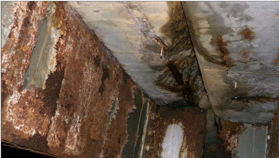
Span 2 Deck: SPALL WITH EXPOSED REBAR TO THE RIGHT SIDE OF BEAM 3 ABOVE BENT 2. UP TO 18 INCHES LONG X 6 INCHES WIDE X 5 INCHES HIGH. EXPOSED REBAR WITH UP TO 70 PERCENT SECTION REMAINING. (PAR)
