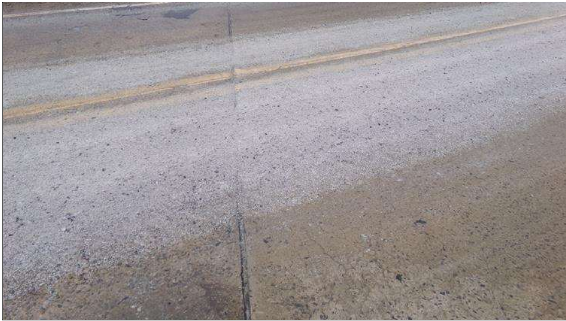
Span 3 Expansion Joint 3: AREAS OF MINOR ADHESION LOSS THRU OUT, MOSTLY CONCENTRATED IN THE SHOULDERS WITH ISOLATED AREAS IN THE ROADWAY
