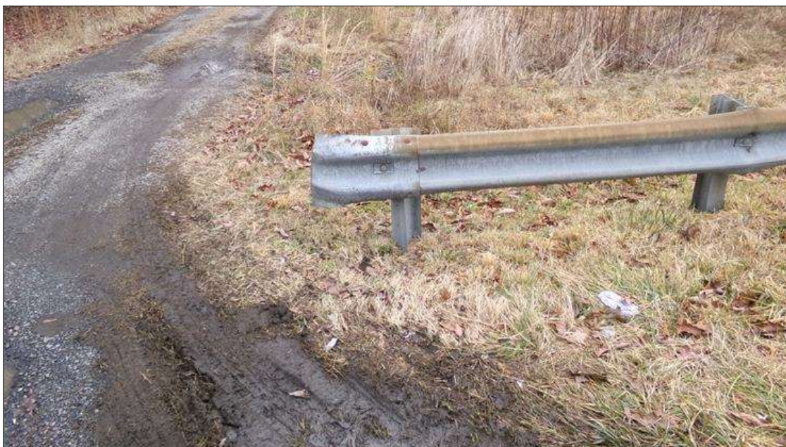
NORTHEAST GUARDRAIL END TERMINAL
