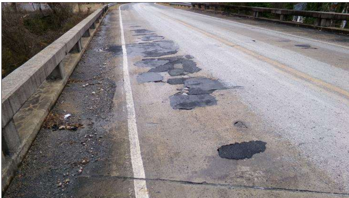
Span 2 Deck: SCATTERED PATCHED AREAS IN TOP OF DECK APPROXIMATELY 20 SQUARE FEET TOTAL
