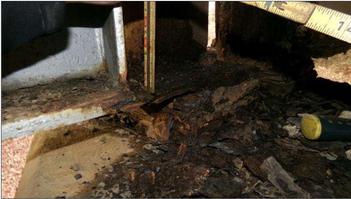
Span 1 Beam 1: WEB SECTION LOSS (33 PERCENT SECTION LOSS, 3/16INCH SECTION LOSS, 3/8INCH REMAINS), 2 INCHES LONG X 8INCHES HIGH AT FAR END (PAR)
