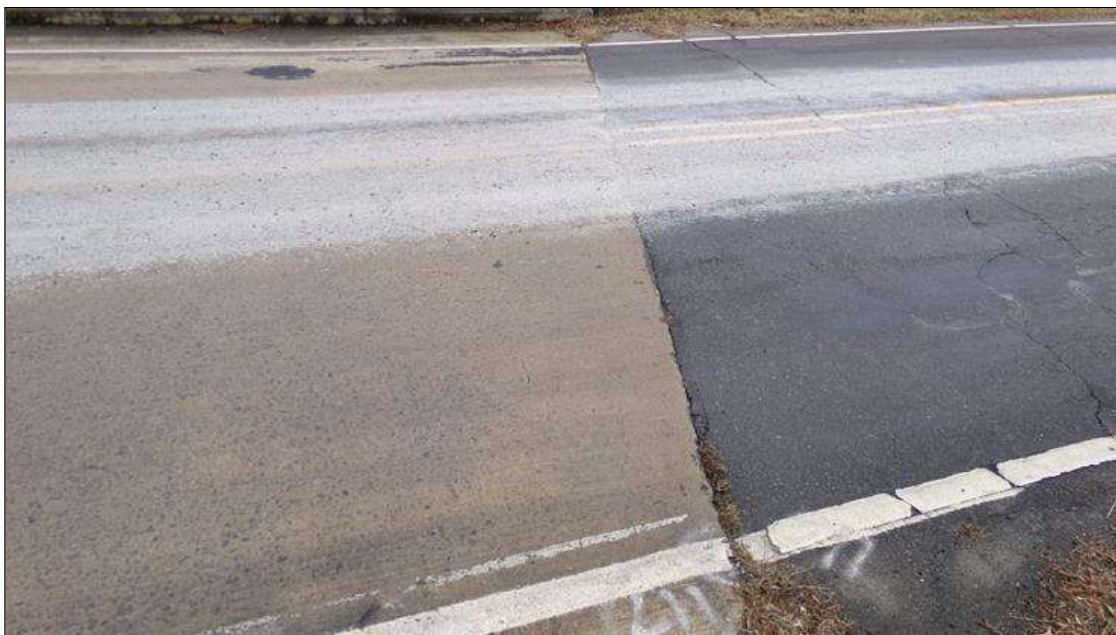
END BENT 1 JOINT, TYPICAL END BENT 2 JOINT
