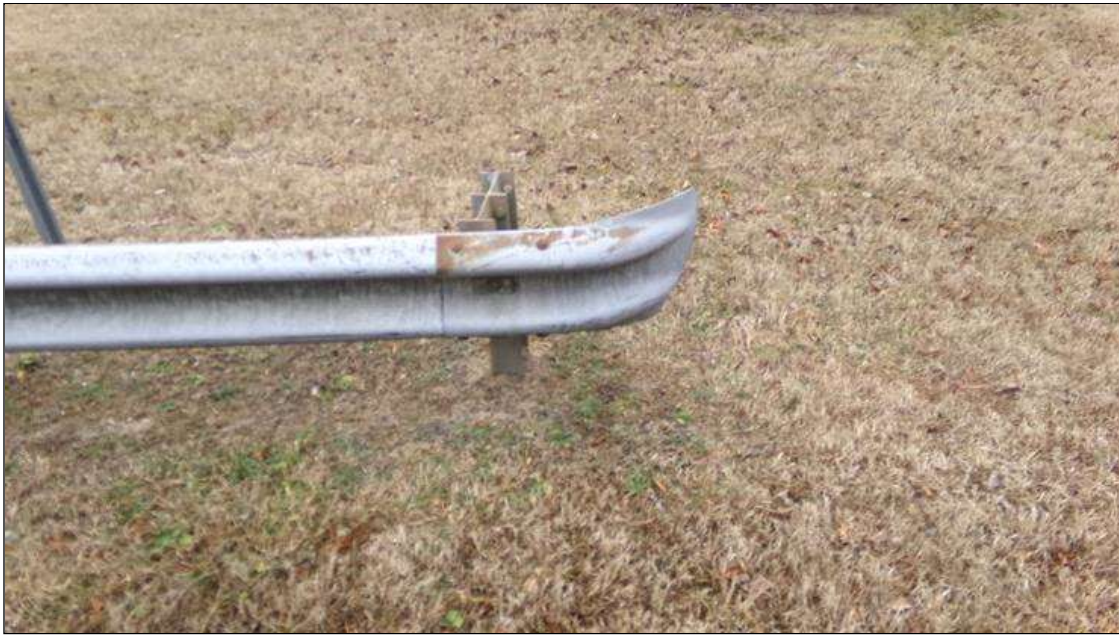
NORTHWEST GUARDRAIL END TERMINAL
