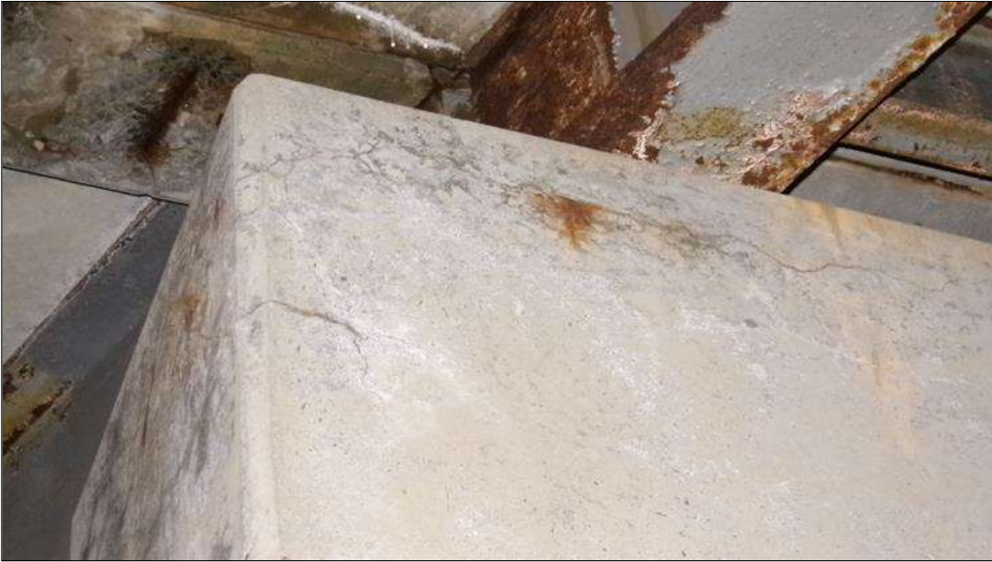
Bent 2 Cap 1: HORIZONTAL OPEN CRACKING (3FEET X 1/8INCH) TOP NEAR FACE AT LEFT END. 5FEET HORIZONTAL OPEN CRACKING (1/16INCH) TO TOP OF CAP UNDER BAY 1. HORIZONTAL OPEN CRACKING (6FEET X 1/8INCH) DELAMINATION TO TOP FAR CORNER AT RIGHT END (DELAMINATION DOES NOT EXTEND UNDER BEARING)
