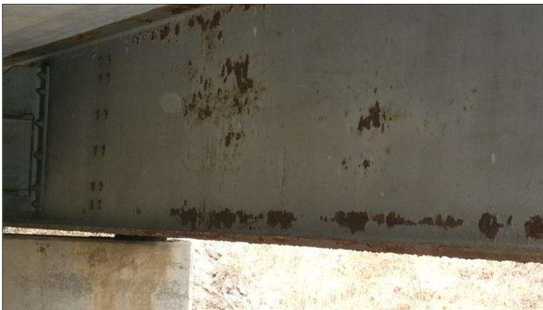
SCATTERED FRECKLED RUST ALONG THE LENGTH OF BEAMS
