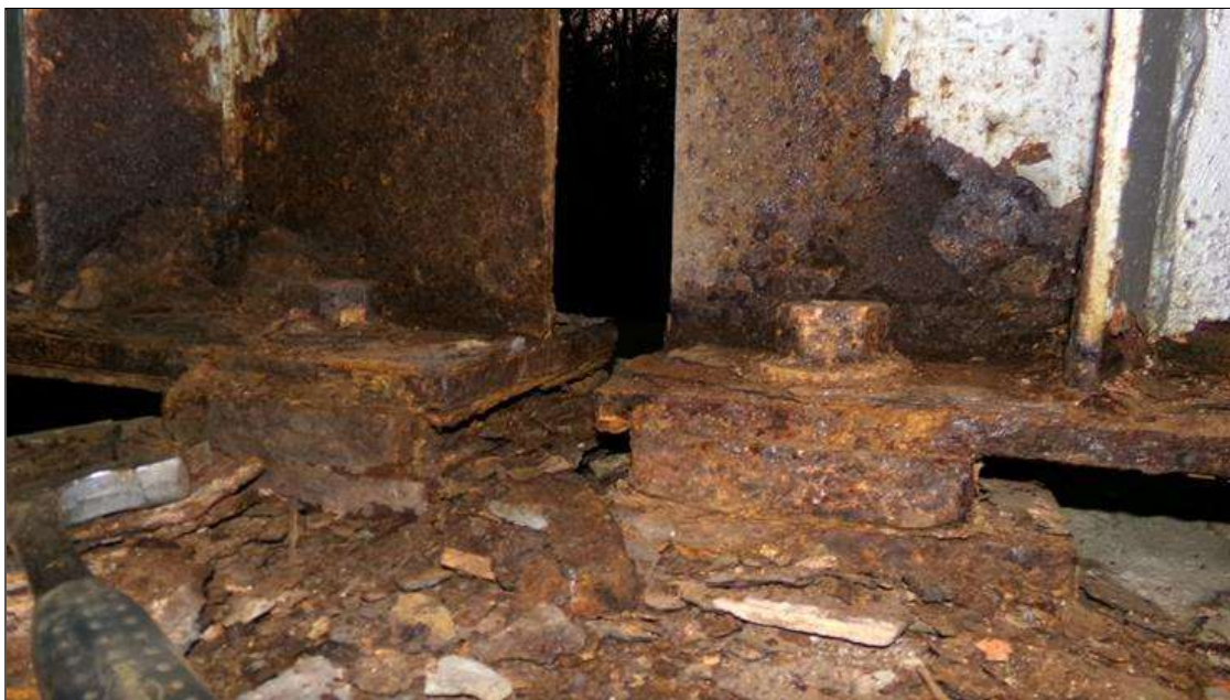
SPAN 2 BEAM 1 FAR BEARING AND SPAN 3 BEAM 1 NEAR BEARING RUST AND SCALE
