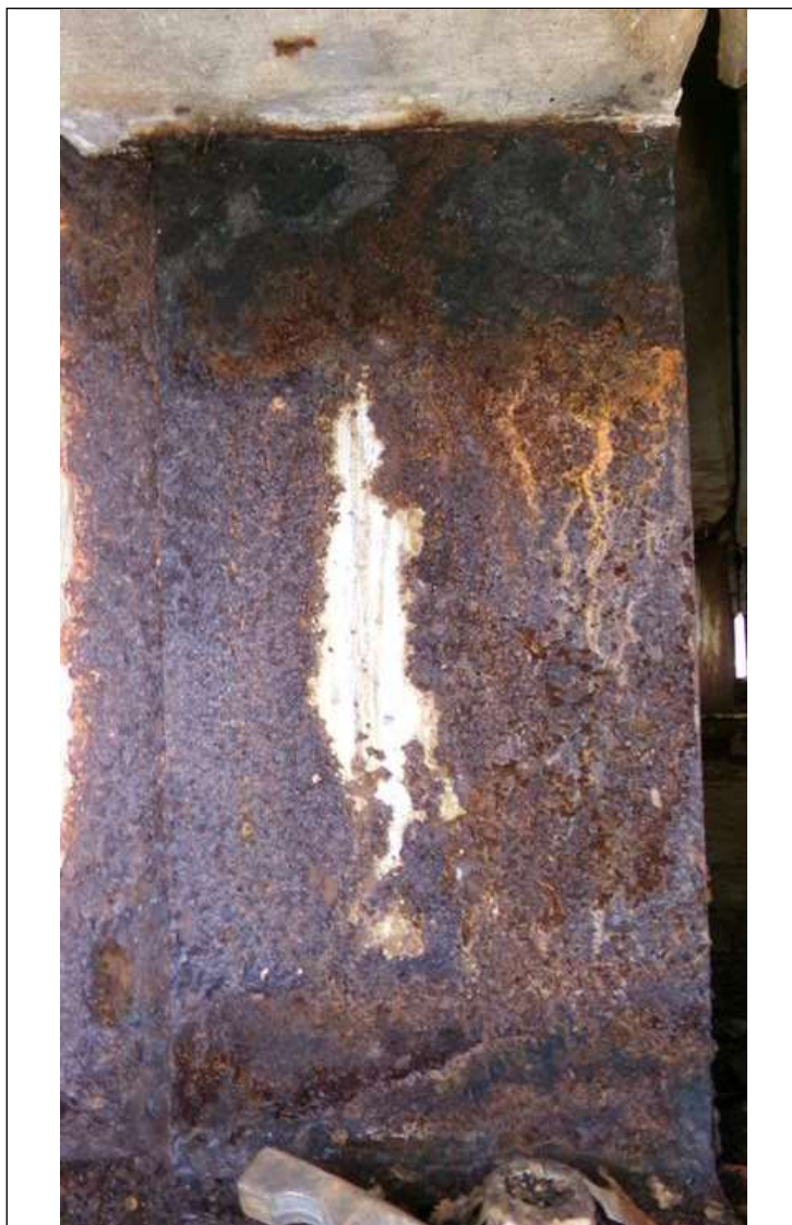
Span 2 Beam 4: WEB PLATE REPAIR (1FOOT X FULL HEIGHT X 1/2INCH THICK) AT FAR END
