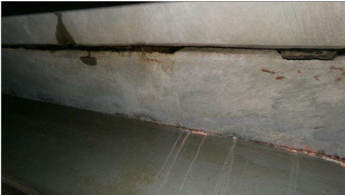
Span 2 Expansion Joint 2: ACTIVE LEAKAGE THROUGH THE JOINT ABOVE BENT IN BAYS 1 AND 3
