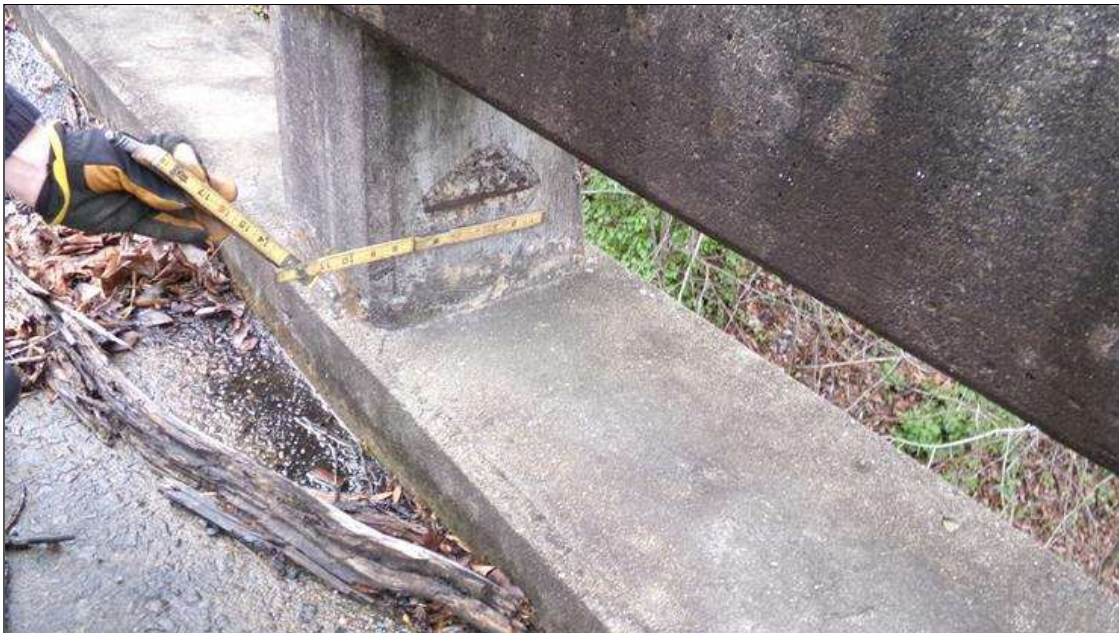
Span 1 Left Bridge Rail: SPALL WITH EXPOSED REBAR UP TO 6 INCHES WIDE X 3 INCHES HIGH X .5 INCHES DEEP IN POST, 8 FEET FROM END OF SPAN.
