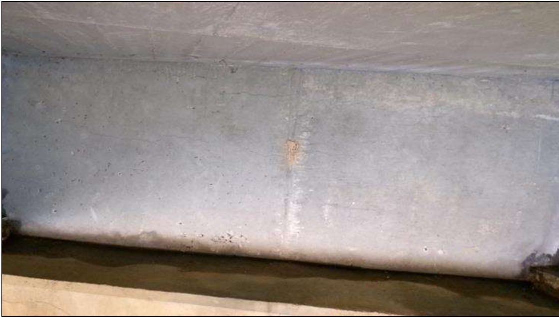
End Bent 1 Abutment: 1FOOT DIAGONAL CRACKING (LESS THAN 1/16INCH) TO ABUTMENT AT FAR ENDS. HORIZONTAL HAIRLINE CRACKING THRU OUT ABUTMENT IN ALL BAYS
