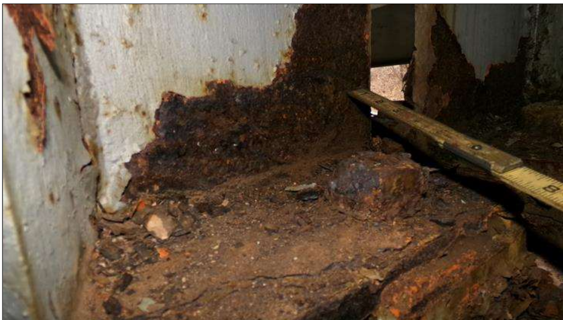
Span 1 Beam 2: BOTTOM FLANGE AND WEB SCALING, 6INCHES HIGH (NO MEASUREABLE SECTION LOSS) FOR 1FOOT AT FAR END.
