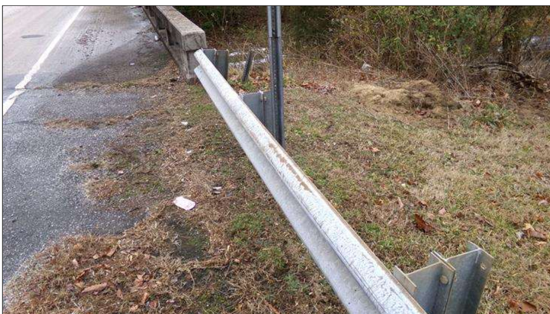
NORTHWEST CORNER GUARDRAIL POST SPACES AT BRIDGE ALL CORNERS SIMILAR
