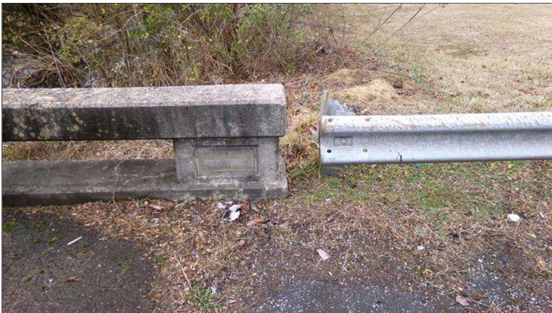
GUARDRAIL DOES NOT ATTACH TO RAIL AT NORTHWEST CORNER
