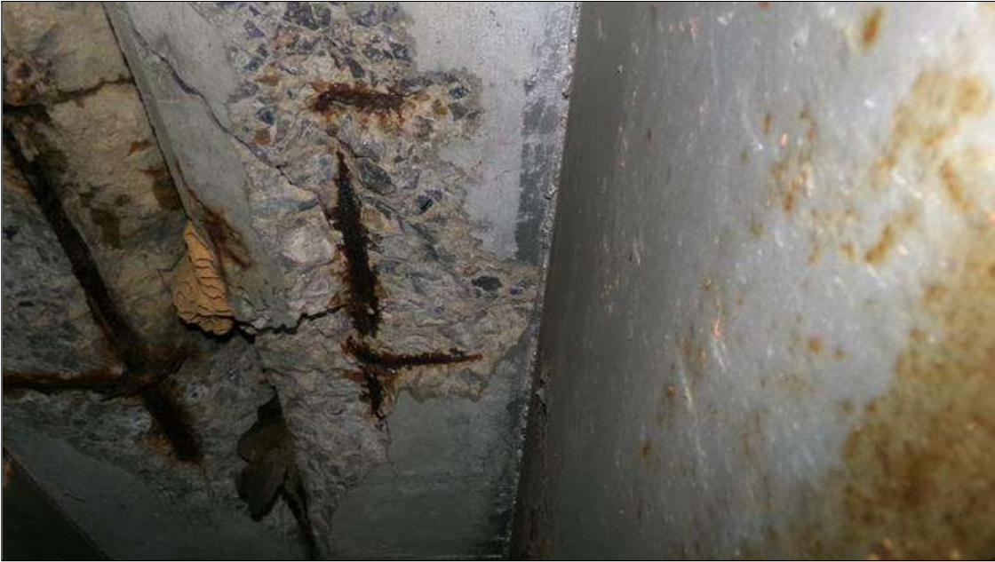
Span 1 Deck: SPALL (3FEET X 10INCHES X 1INCH SPALL) WITH EXPOSED SCALING TO REBAR TO BOTTOM OF DECK IN BAY 2 OVER BENT 1. UP TO 90 PERCENT SECTION REMAINING IN THE EXPOSED REBAR (PAR)
