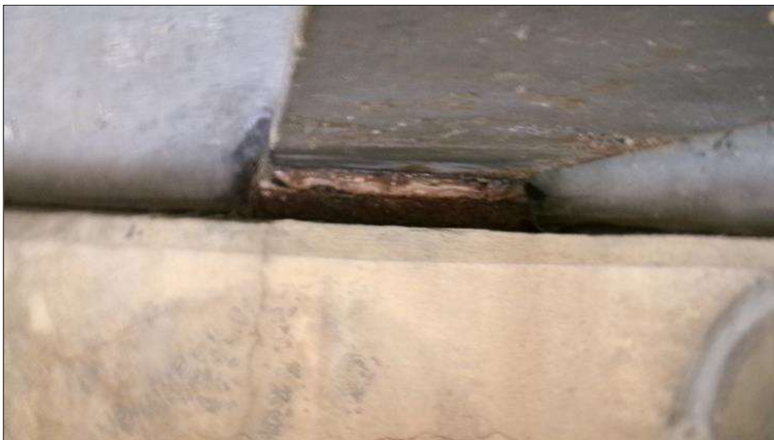
TYPICAL BEARING AT END BENT 1
