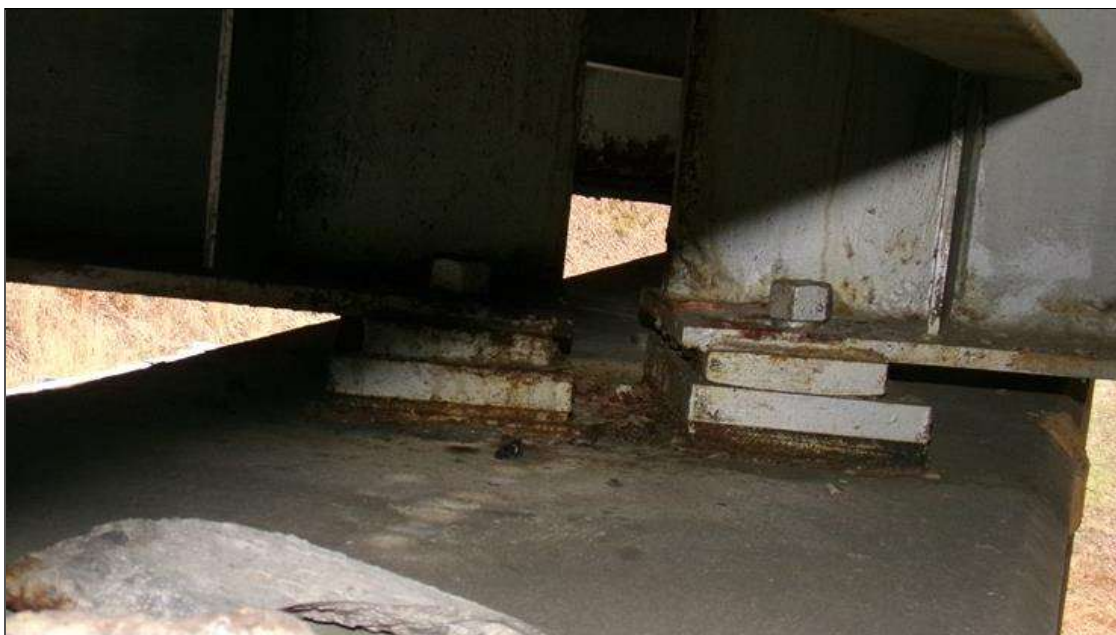
TYPICAL BEARING AT BENT 1 SPANS 1 AND 2 BEAM3
