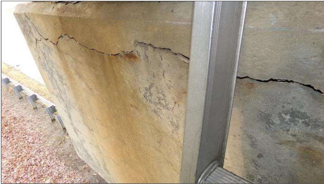
Bent 1 Cap 1: HORIZONTAL OPEN CRACKING (UP TO 5 FEET X 1/8 INCH) AND 3 FEET DELAMINATION TO NEAR AND FAR FACES AT TOP OF CAP AT RIGHT AND LEFT ENDS. (DELAMINATION DOES NOT EXTEND UNDER BEARING)
