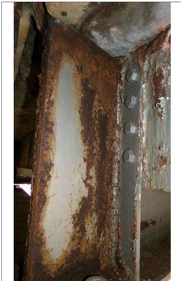
Span 2 Beam 3: WEB PLATE REPAIR LEFT SIDE (1FOOT X FULL HEIGHT X 1/2INCH THICK) AT FAR END
