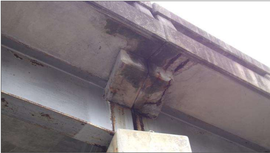
Span 1 Deck: SPALL AND DELAMINATION (UP TO 3FEET X 20INCHES X 1INCH) WITH EXPOSED SCALING REBAR TO LEFT OVERHANG AT FAR END. UP TO 90 PERCENT REMAINING IN THE EXPOSED REBAR. (PAR)
