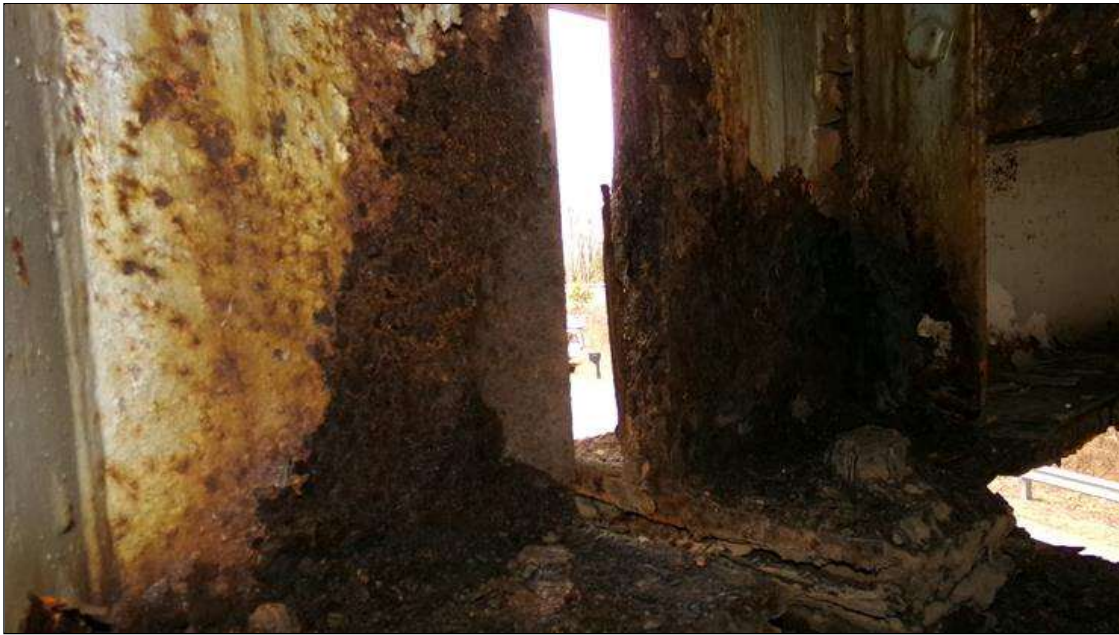
Span 2 Beam 1: WEB SCALING AT BEAM FAR AND NEAR ENDS FOR FULL HEIGHT UP TO 1/16 INCH LOCALIZED SECTION LOSS (1/2 INCH REMAINS) AT BOTTOM FOR 2 INCH HIGH
