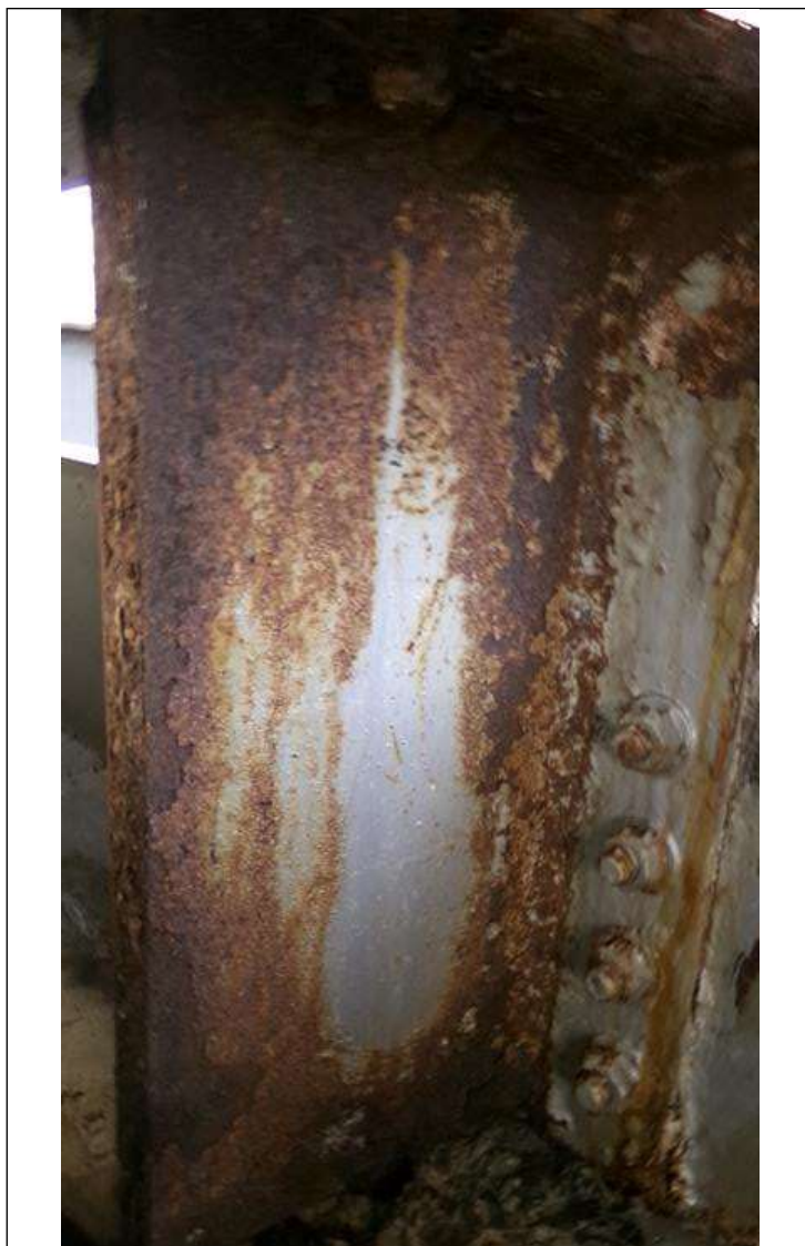
Span 2 Beam 3: WEB PLATE REPAIR RIGHT SIDE (1FOOT X FULL HEIGHT X 1/2INCH THICK) AT FAR END
