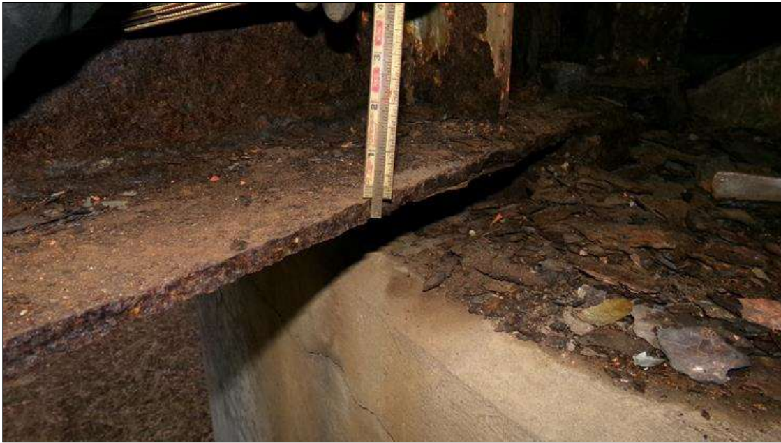
Span 3 Beam 4: BOTTOM FLANGE SECTION LOSS (33 PERCENT SECTION LOSS, 1/4INCH SECTION LOSS, 7/16INCH REMAINS) FULL WIDTH AND WEB PITTING (1/2INCH REMAIN X 4INCHES HIGH) FOR 5FEET AT NEAR END. LEFT STIFFENER HAS UP TO 1/8 INCH SECTION LOSS FOR 3 INCHES HIGH X FULL WIDTH (PAR)
