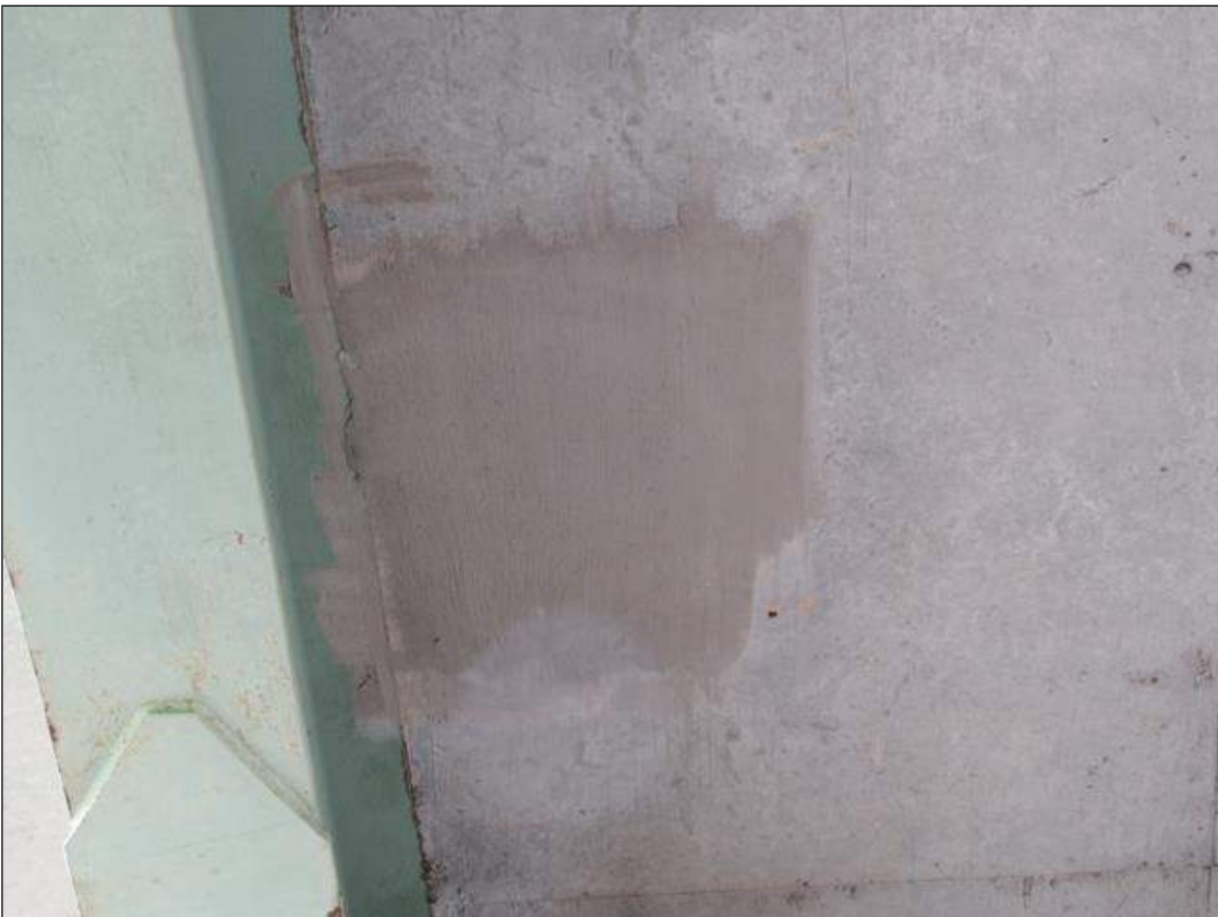
Span 2 Deck: UNDERSIDE OF DECK, SOUND PATCH, BAY 1 RIGHT OF BEAM 1, MID SPAN
