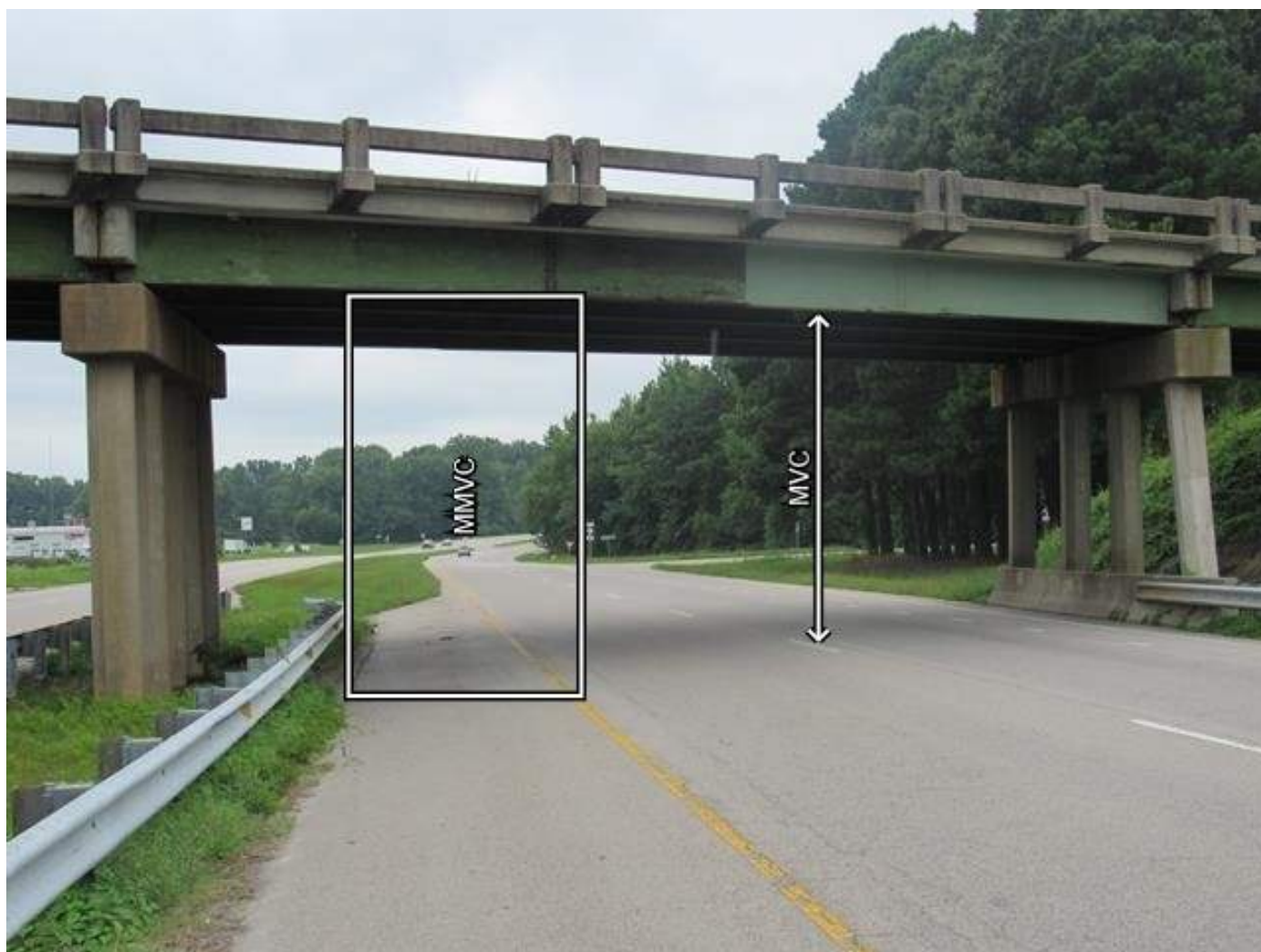
SPAN 2 CLEARANCE OPENING LOOKING SOUTH
