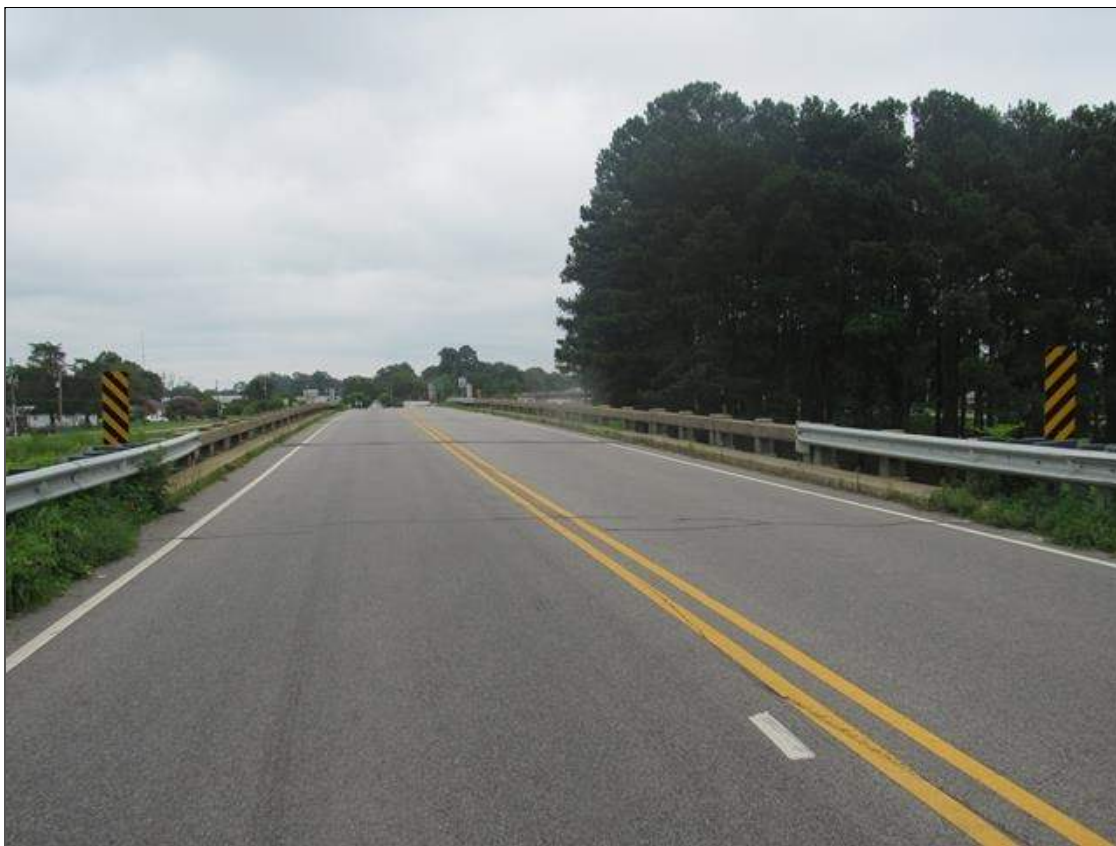
WEST APPROACH LOOKING EAST
