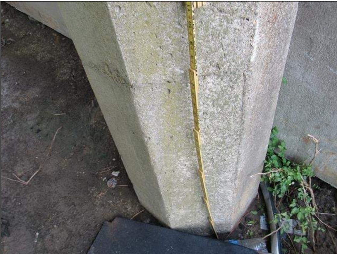
Bent 3 Pile 1: HAIRLINE MAP CRACKING ON NORTHEAST CORNER (2 FOOT HEIGHT), BASE OF PILE
