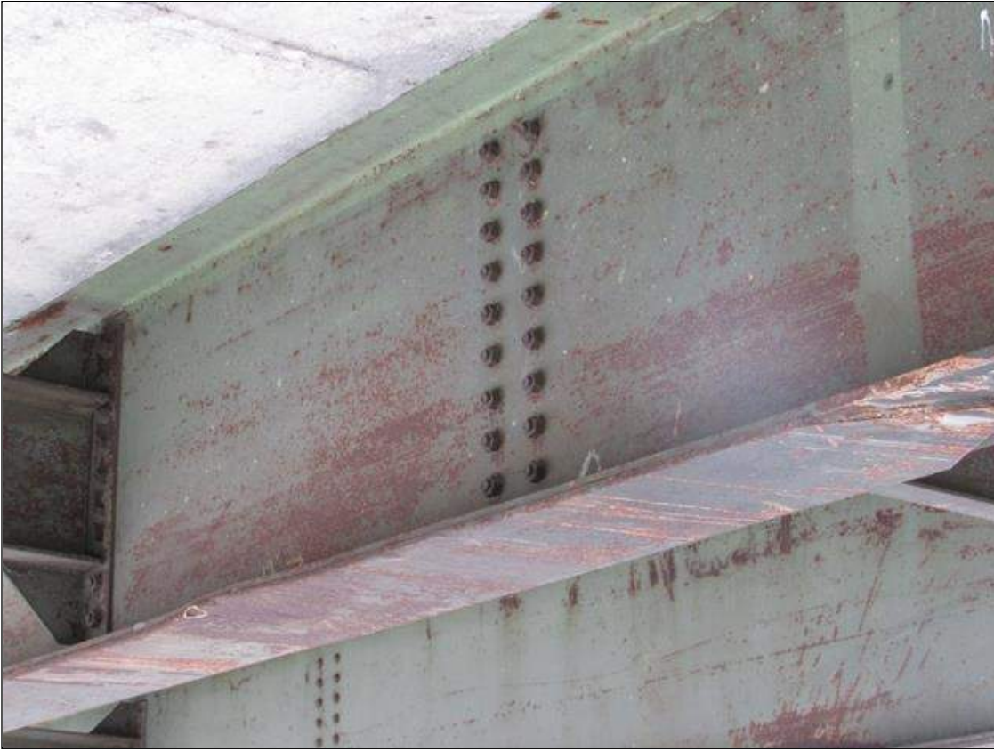
Span 3 Beam 3: 1 1/2 INCH LONG X 3/16 INCH DEEP GOUGE IN BOTTOM FLANGE COVER PLATE TO BEAM, BEAM IS BOWED UPWARDS 1/2 INCH FOR A LENGTH OF 2 FOOT 6 INCH LONG LOCATED 19 FEET FROM EAST END OF BEAM (PAR)
