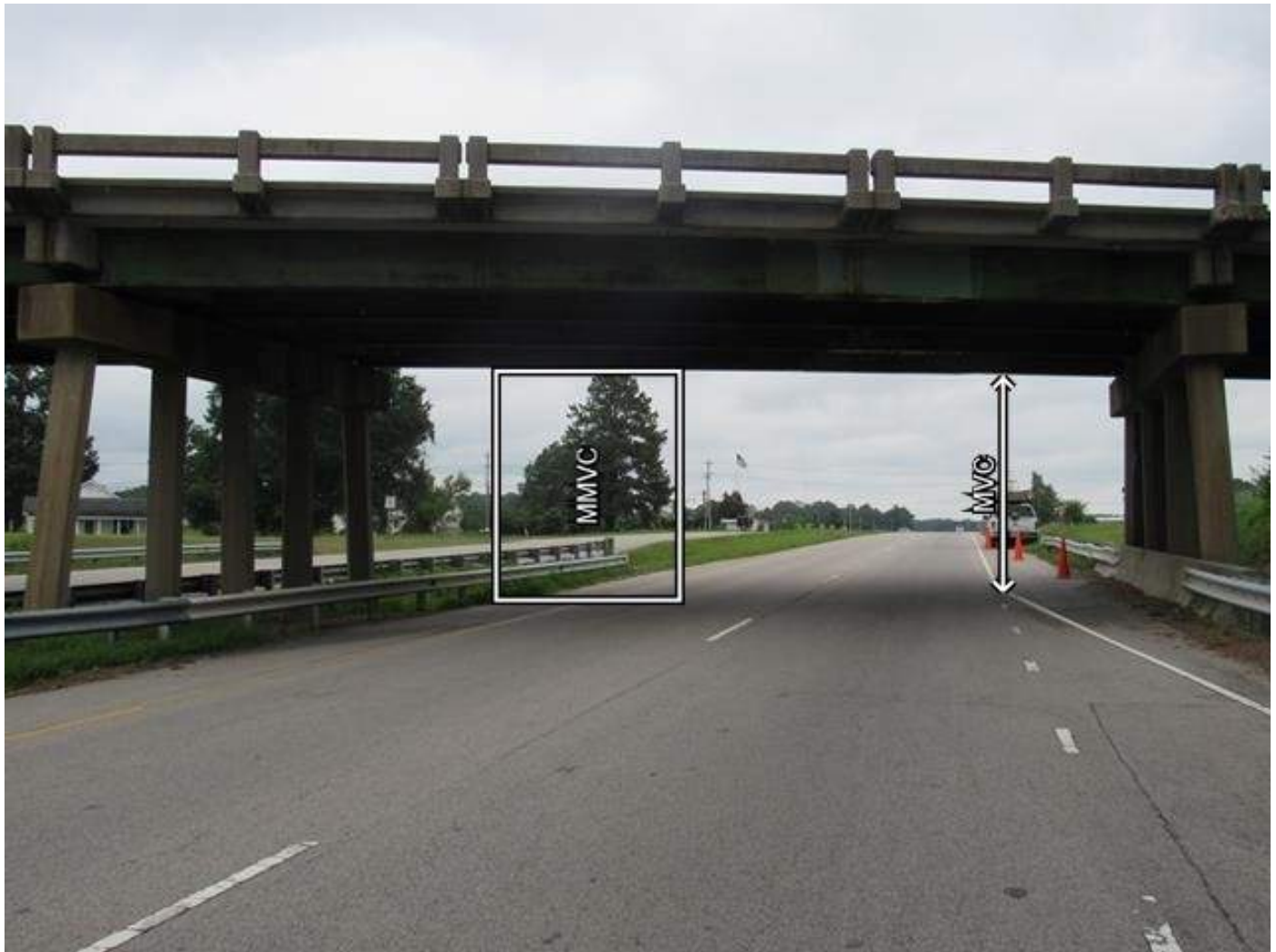
SPAN 3 CLEARANCE OPENING LOOKING NORTH
