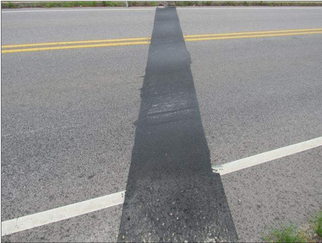
WEARING SURFACE OVER BENT 1
