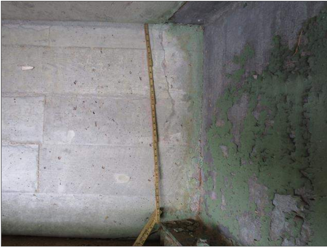
End Bent 2 Abutment: 1 FOOT 6 INCH HIGH X 9 INCH WIDE AREA OF DELAMINATION ADJACENT TO LEFT TOP FLANGE OF BEAM 3, 2 FOOT 9 INCH HIGH X 9 INCH WIDE AREA OF DELAMINATION ADJACENT TO RIGHT TOP FLANGE OF BEAM 3
