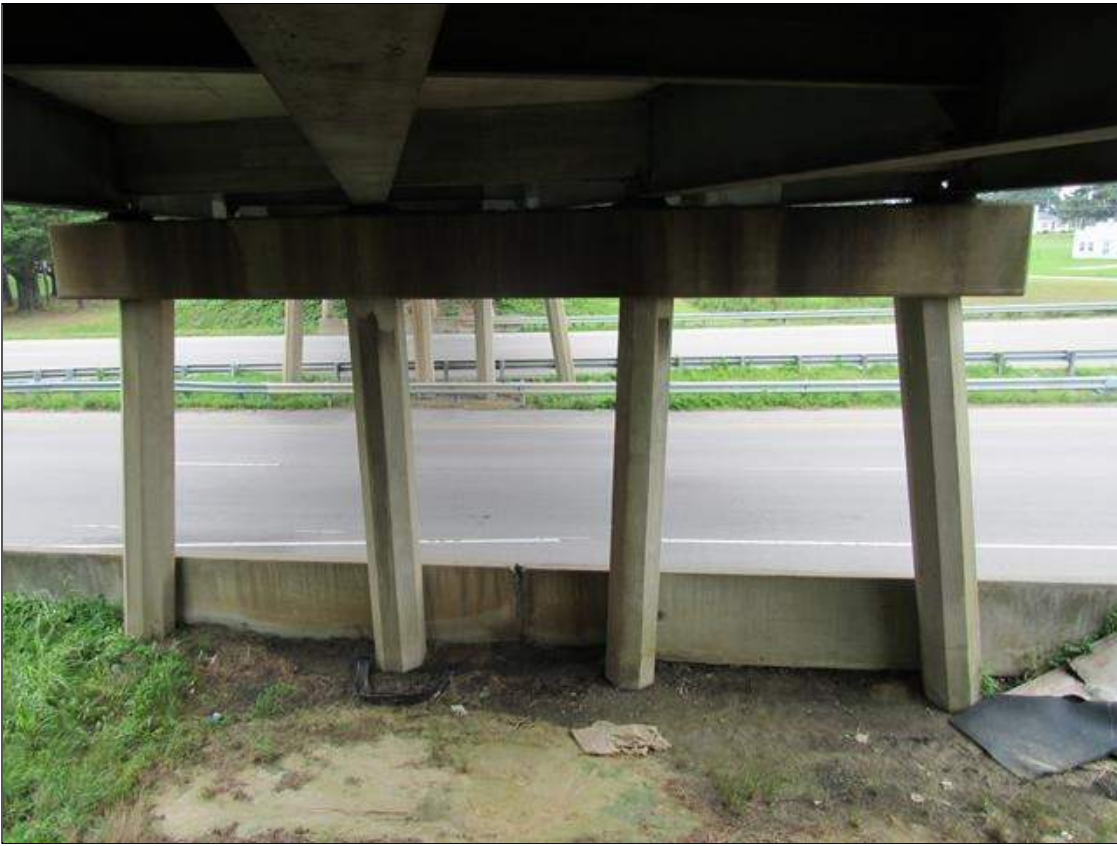
BENT 3 LOOKING WEST
