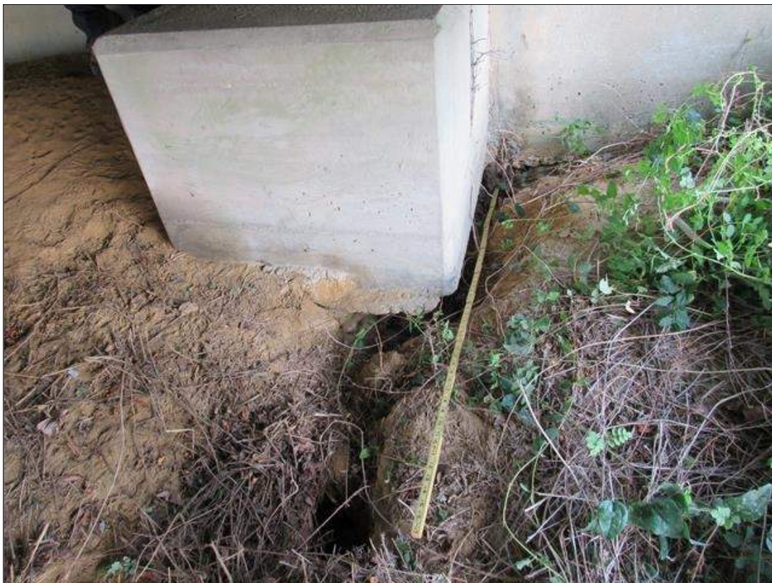
AREA OF EROSION 22 INCH WIDE X 6 FEET LONG X UP TO 9 INCHES DEEP UNDER LEFT BRACE PILE AT END BENT 1, BRACE PILE CAP IS UNDERMINED AND PILE IS EXPOSED UP TO 9 INCHES (PAR)
