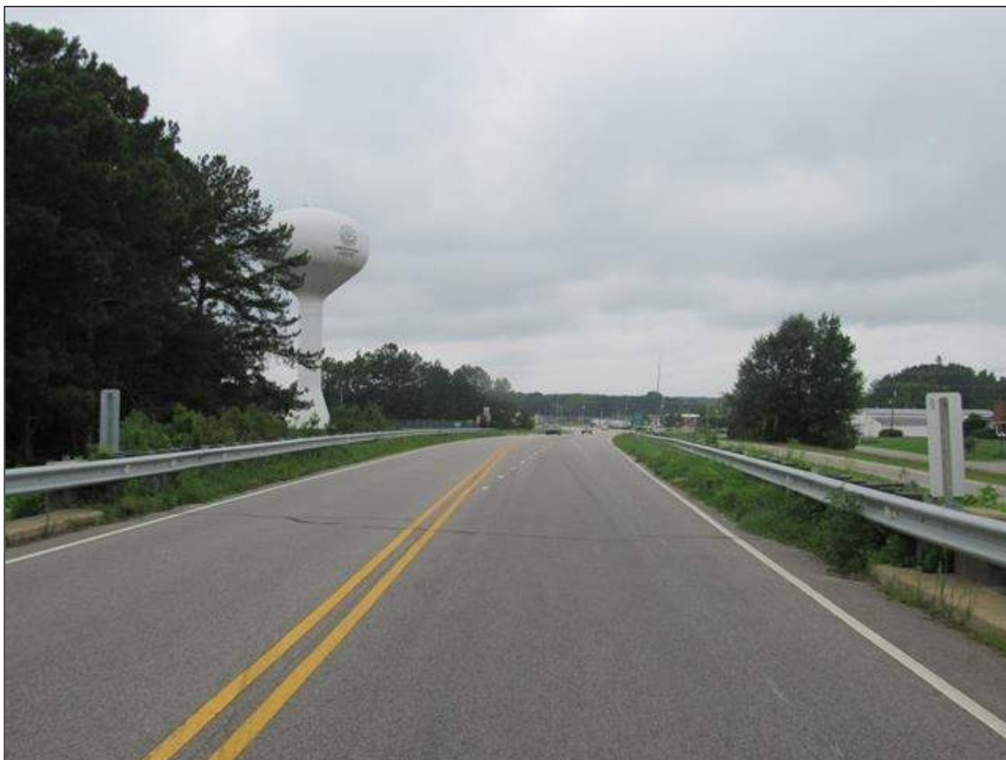
WEST APPROACH LOOKING WEST
