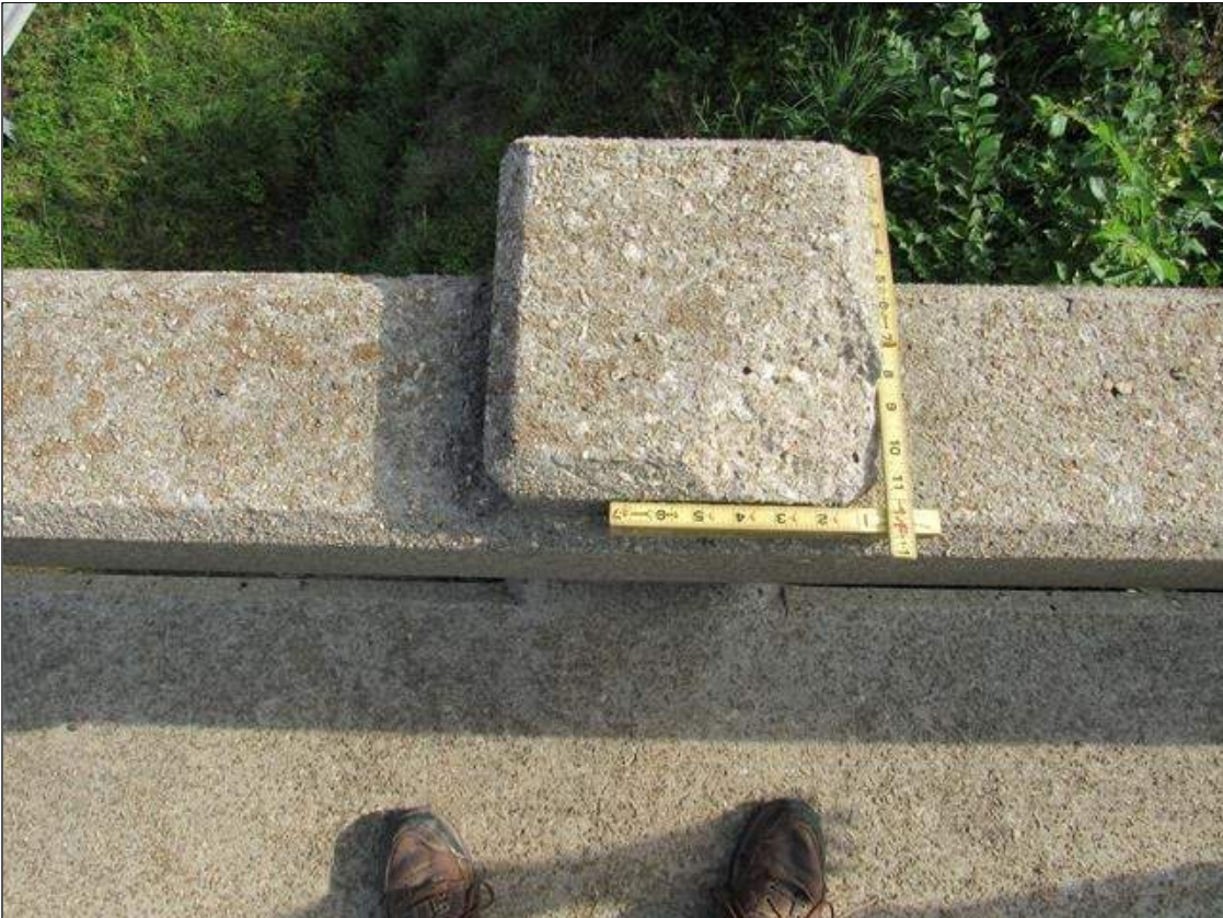
Span 4 Left Bridge Rail: 5 INCH LONG X 5 INCH WIDE X 1 INCH DEEP SPALL ON TOP OF POST 5 (SAME ON POST 8)
