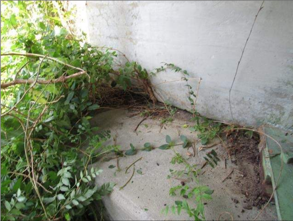
VEGETATION GROWING BETWEEN END BENT 1 CAP AND BACKWALL AT SOUTH END
