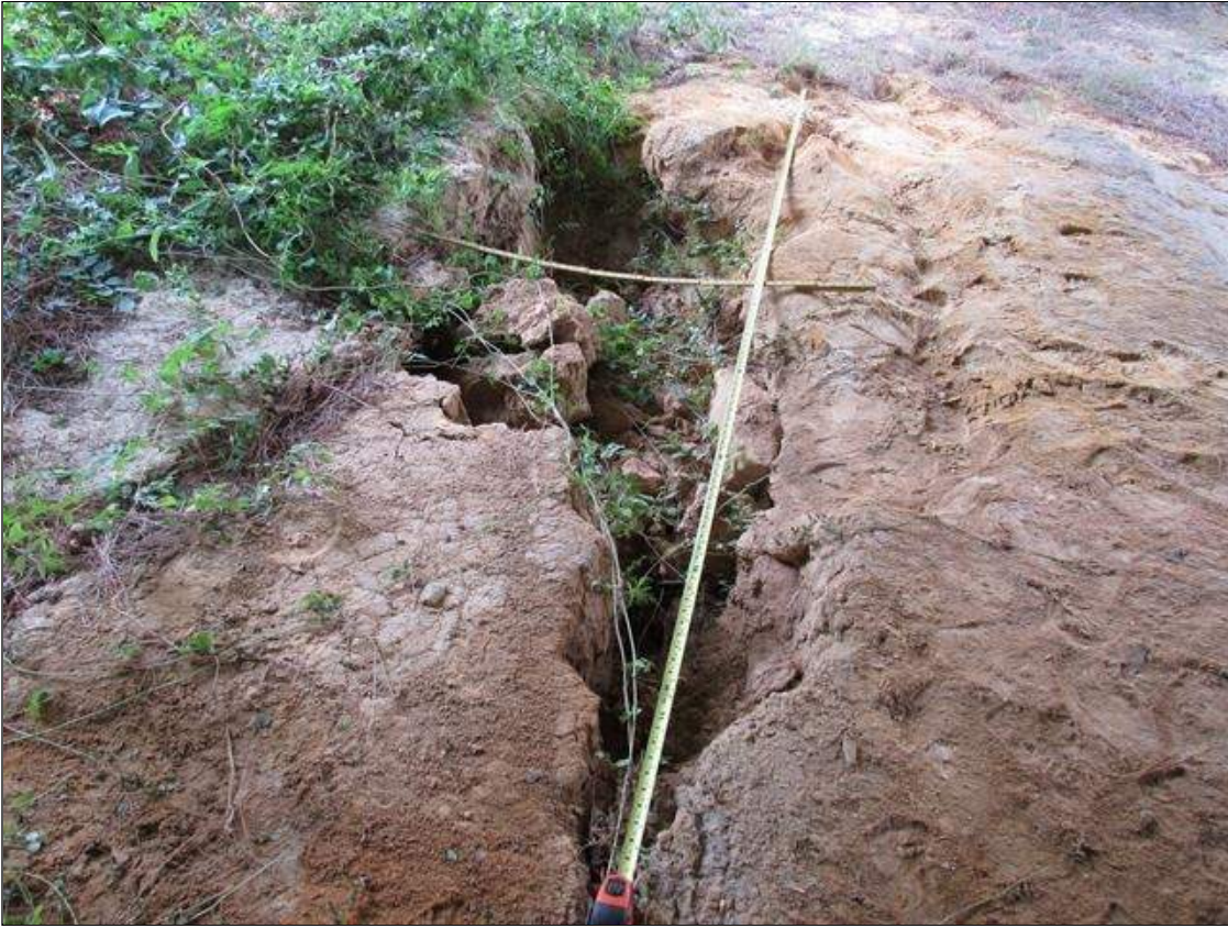
AREA OF EROSION 11 FOOT LONG X 4 FOOT WIDE X UP TO 2 FOOT DEEP AT END BENT 2 UNDER BAY 3 (PAR)
