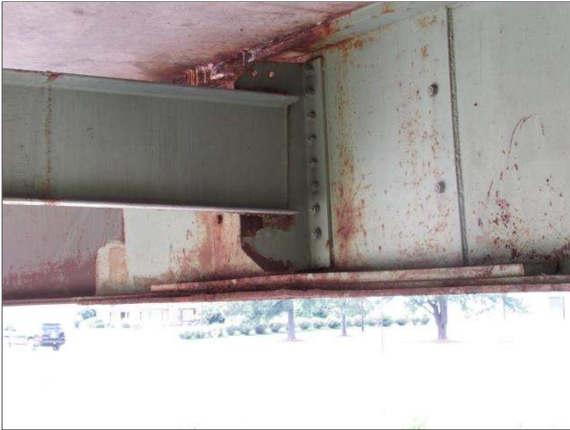
Span 3 Beam 1: BOTTOM FLANGE OF BEAM 1 IN SPAN 3 IS BOWED UPWARDS 1/2 INCH FOR A LENGTH OF 4 FEET OVER RIGHT LANE (PAR)
