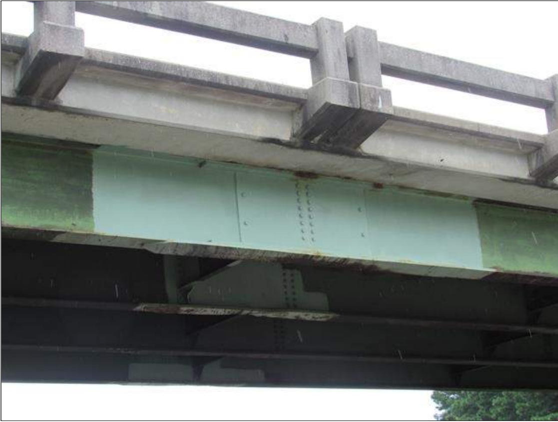
SPAN 3 BEAM 1 REPAIR
