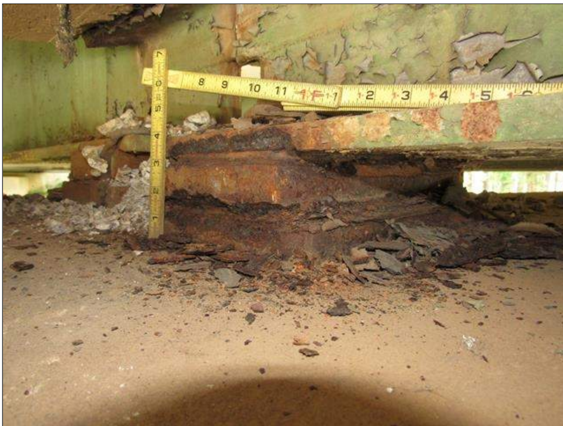
Span 3 Beam 3 - Far Bearing: PACK RUST AND HEAVY CORROSION, SECTION LOSS HAS INITIATED
