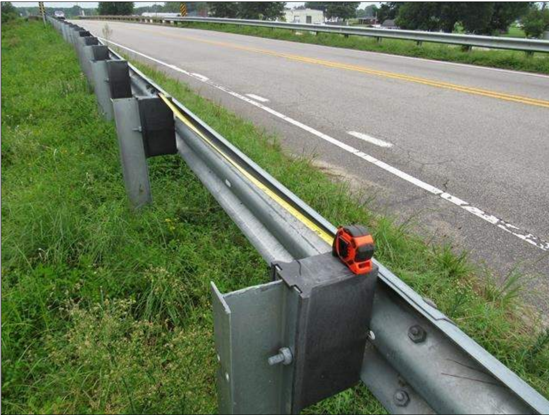
TYPICAL GUARDRAIL POST SPACING 6.25 FEET (SOUTHEAST SHOWN, ALL OTHERS SIMILAR)
