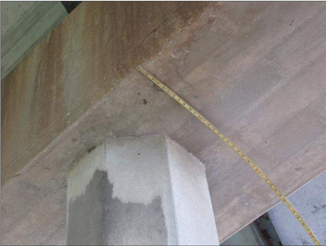
Bent 3 Cap 1: 0.007 INCH WIDE X FULL-WIDTH TRANSVERSE CRACK IN UNDERSIDE OF CAP LEFT OF PILE 3
