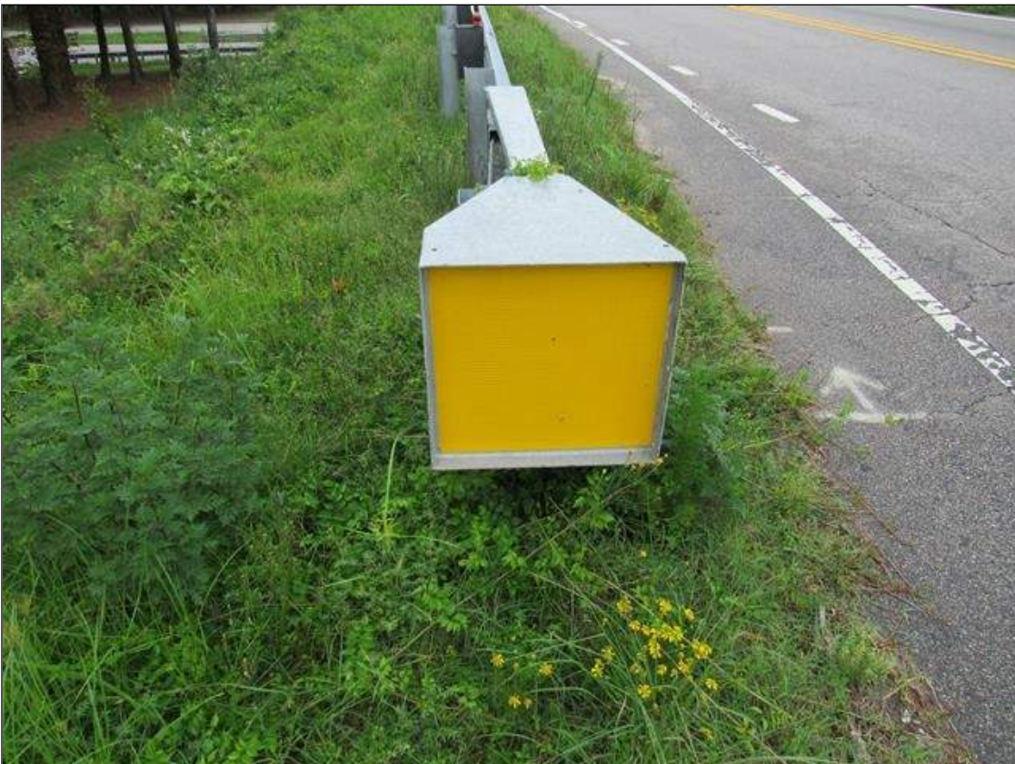
TYPICAL GUARDRAIL END TERMINAL (SOUTHEAST SHOWN, ALL OTHERS SIMILAR)
