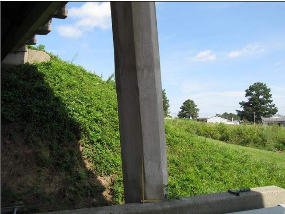
Bent 1 Pile 1: 22 INCH X 8 INCH X 1 INCH DEEP SPALL WITH EXPOSED REBAR ON EAST FACE AT BARRIER RAIL -DEFECT HAS BEEN REPAIRED WITH A SOUND PATCH AS OF 8/18/2022 (SEE PHOTO)
