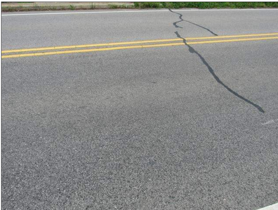
WEARING SURFACE OVER END BENT 1
